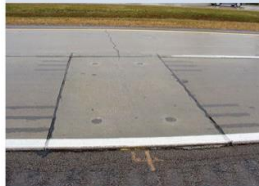
Dowel bars fabricated in precast panel
