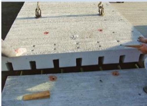
Dowel bars drilled in existing slab
