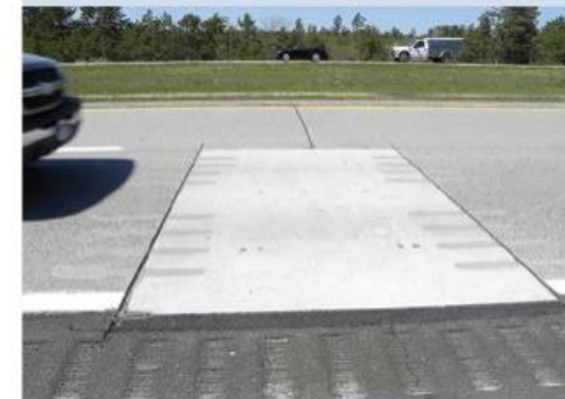
Precast panel using full dowel bar retrofit installation
