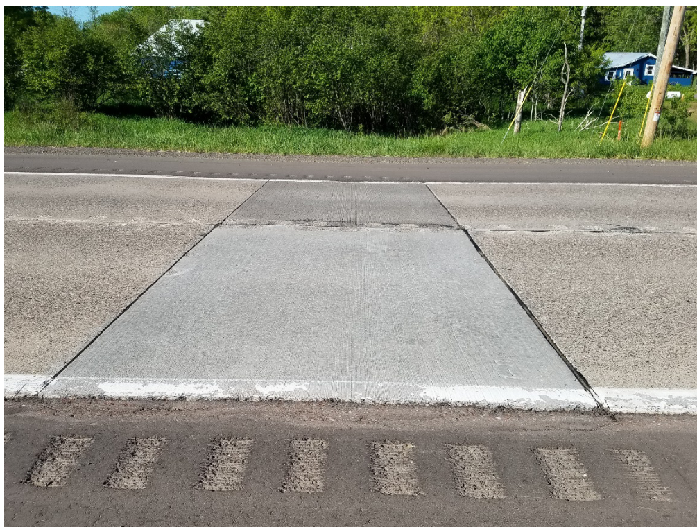
Figure 9-7. Typical full-depth joint repair.
