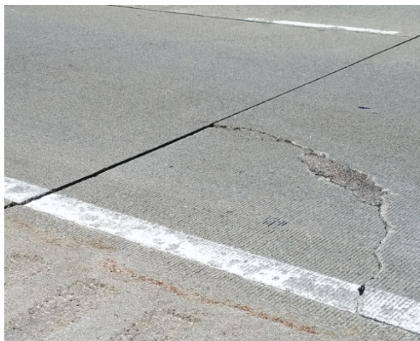
Figure 3-7. Example of medium-severity, mid-panel crack (left image) and corner break (right image) in 2018.
