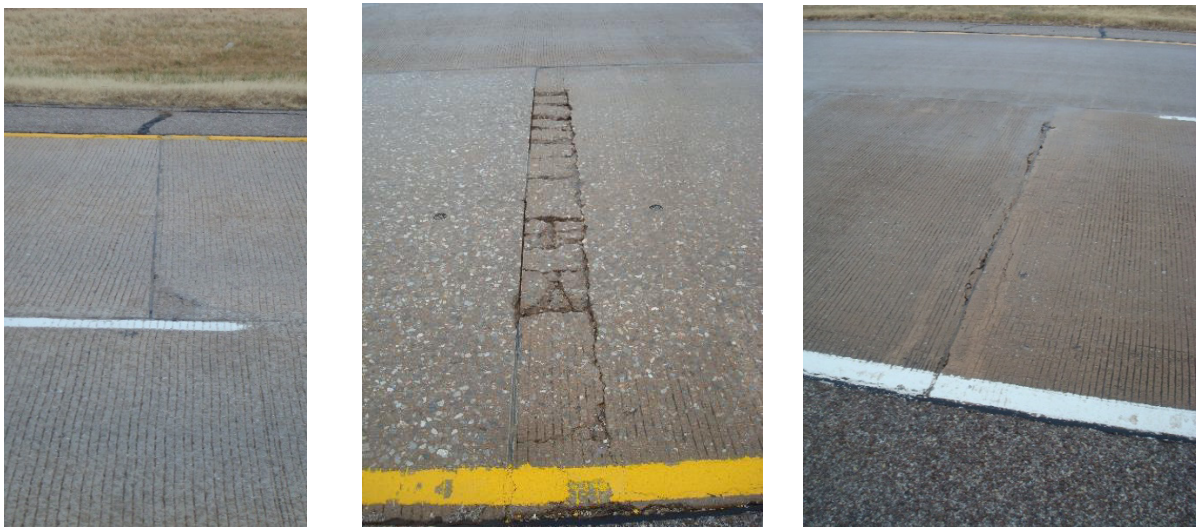
Figure 7-14. Examples of overlay deterioration around transverse construction joints.
