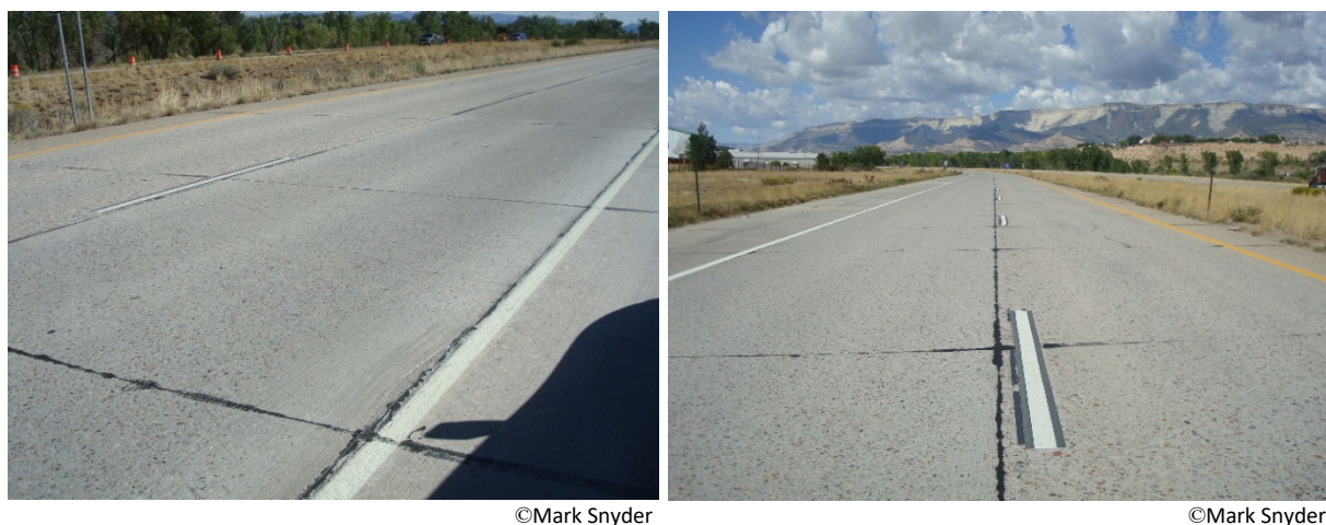
Figure 10-8. Examples of typical good overall pavement condition.
