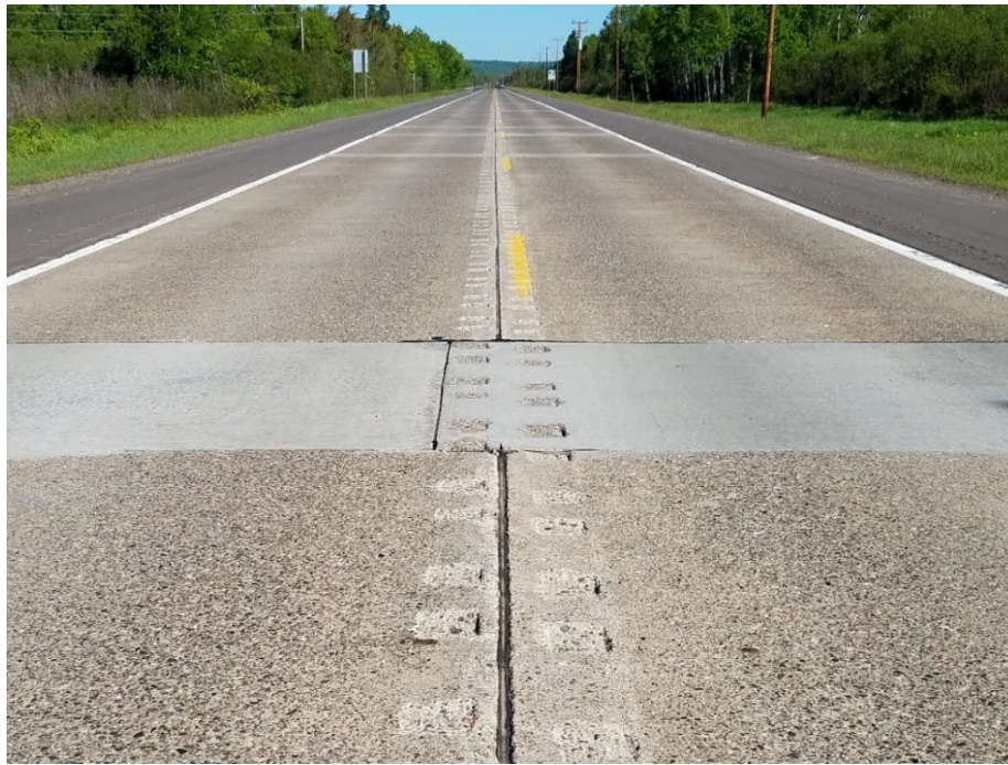
Figure 9-4. View of the project showing full-depth repairs and worn concrete surface.
