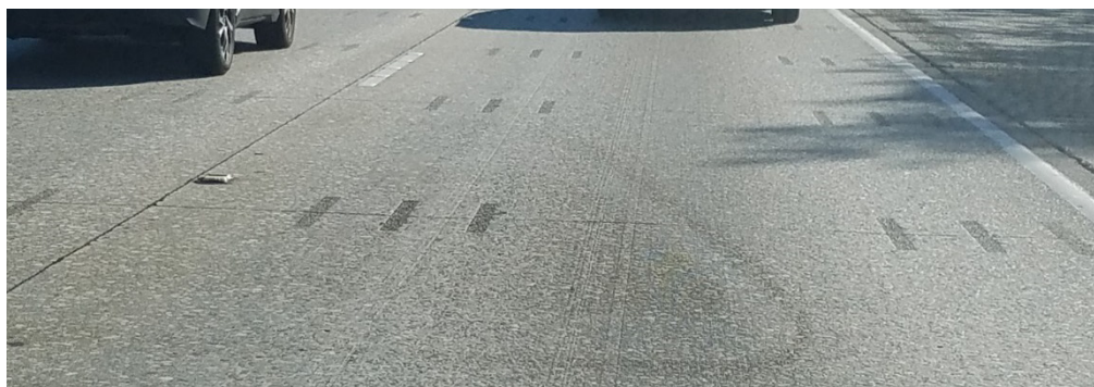
Figure 12-4. View of the northbound project showing dowel bar retrofitting and texture produced by diamond grinding in outer (truck) lane) constructed in 1996.
