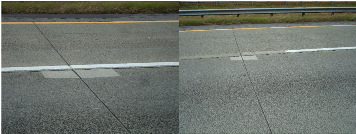
Figure 5-9. Typical partial-depth joint spall repairs on NC I-85 overlay project.
