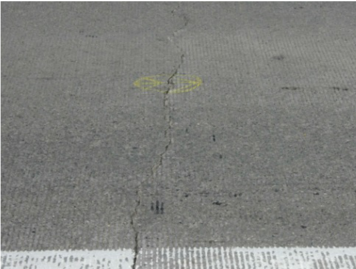
Figure 3-5. Low- to medium-severity transverse cracking in 2011.
