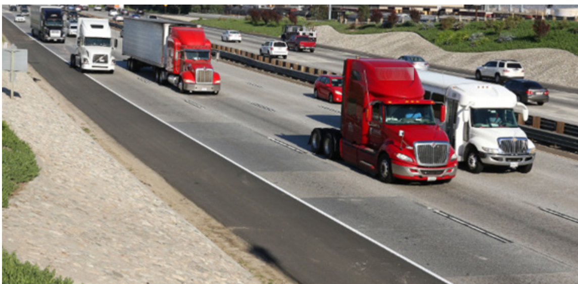
Figure 11-4. Example view of existing concrete pavement in 2017 showing replaced slabs. Left two lanes (in photo) are original concrete pavement.
