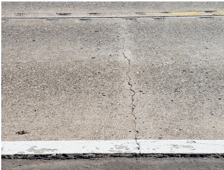
Figure 9-5. Low-severity mid-panel crack.
