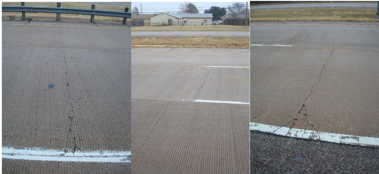
Figure 7-11. Typical wide (deteriorating) transverse cracks.
