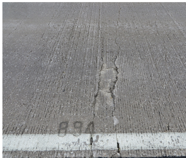
Figure 4-7. Spalling along transverse crack (left) and punchout (right).
