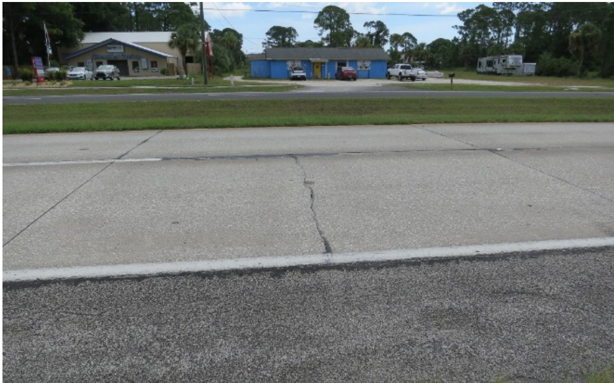
Figure 6-4. Example transverse cracking on 20-ft panel observed in 2018.
