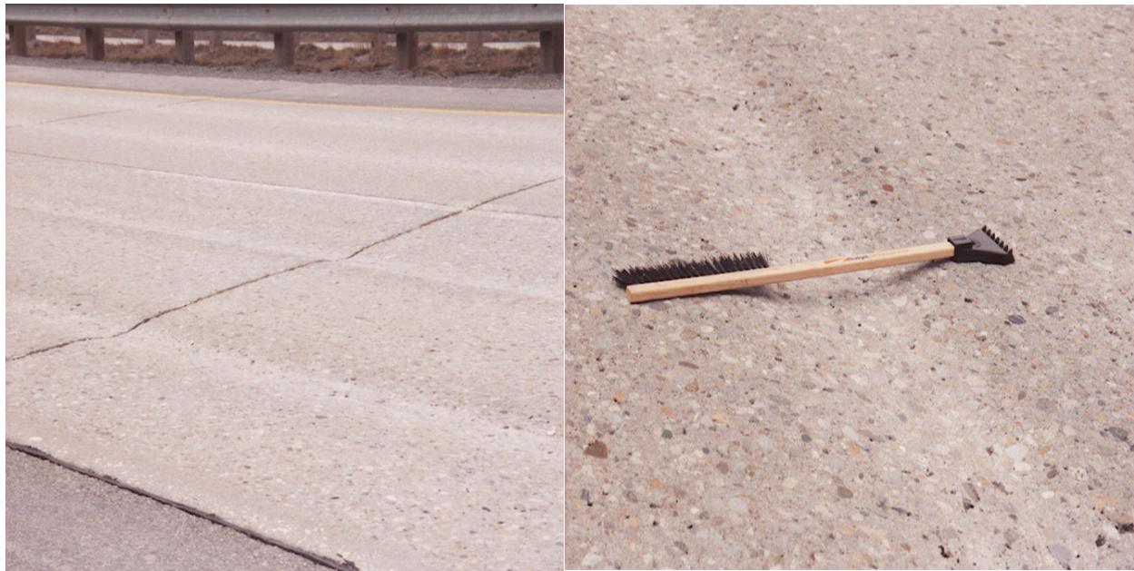
Figure 10-4. Project wheel path rutting due to tire chains and studded tires (Necessary and Lemasany 2006).
