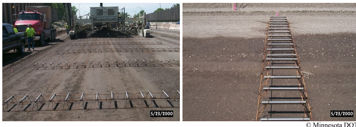
Figure 2-2. Dowel bar configuration used in the I-35W project.
