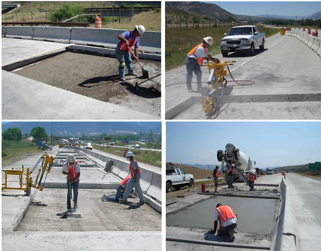
Figure 10-5. 2005 full-depth repair construction (Necessary and Lemasany 2006).
