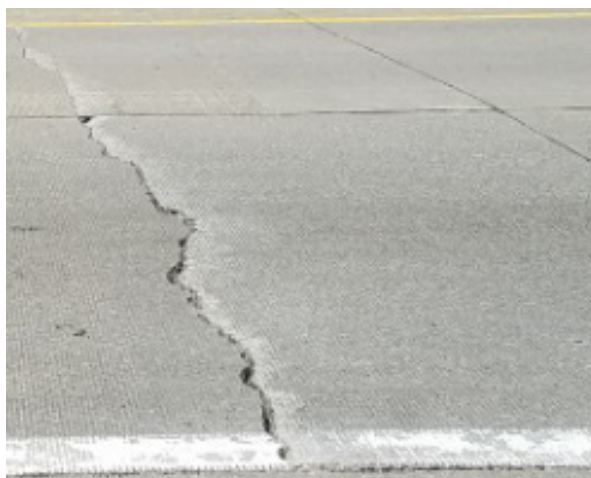
Figure 3-7. Example of medium-severity, mid-panel crack (left image) and corner break (right image) in 2018.
