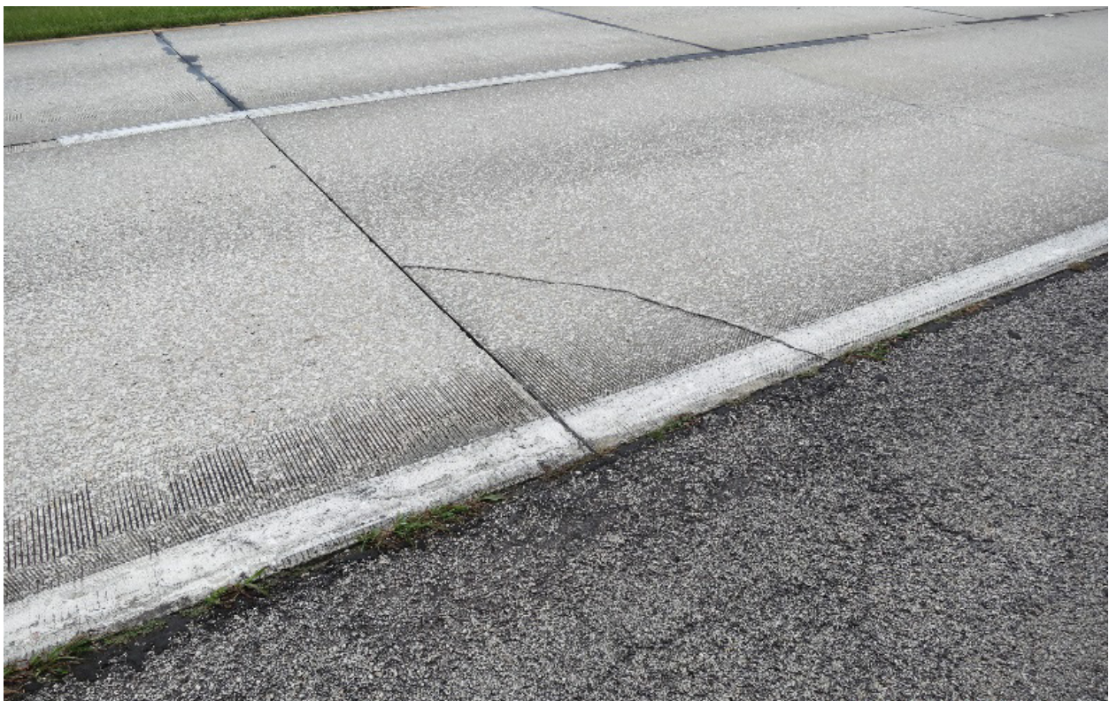
Figure 6-6. Corner break on control section in 2018.
