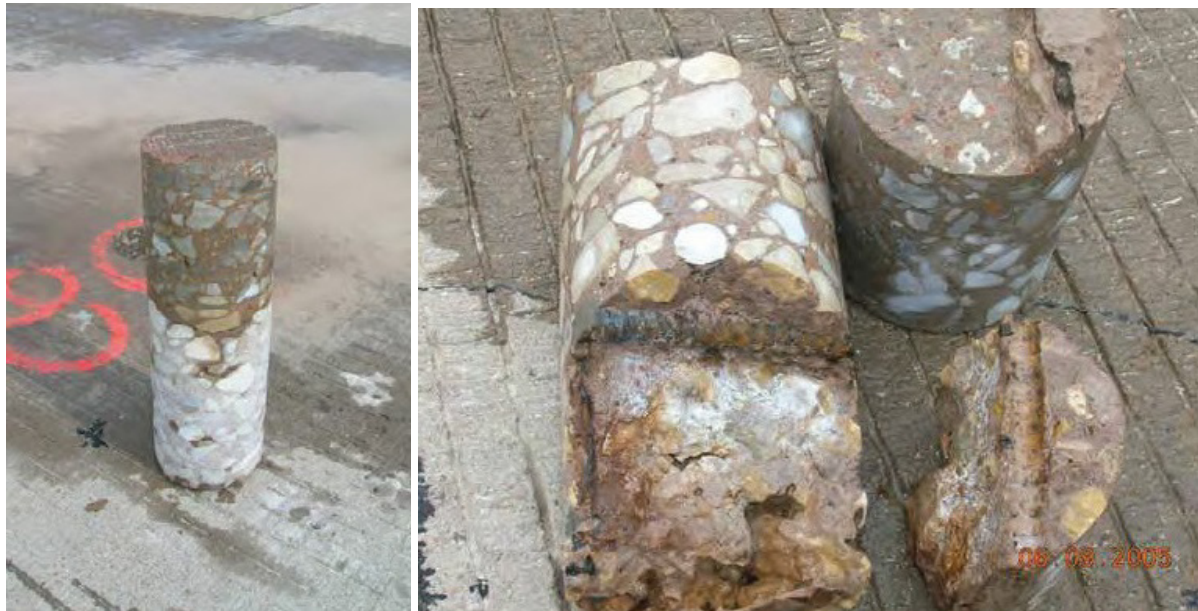
Figure 7-6. Photos of typical U.S.-281 core in good condition (left) and deteriorated and delaminated core (right). (Trevino, Medina-Chavez, and Won 2005)
