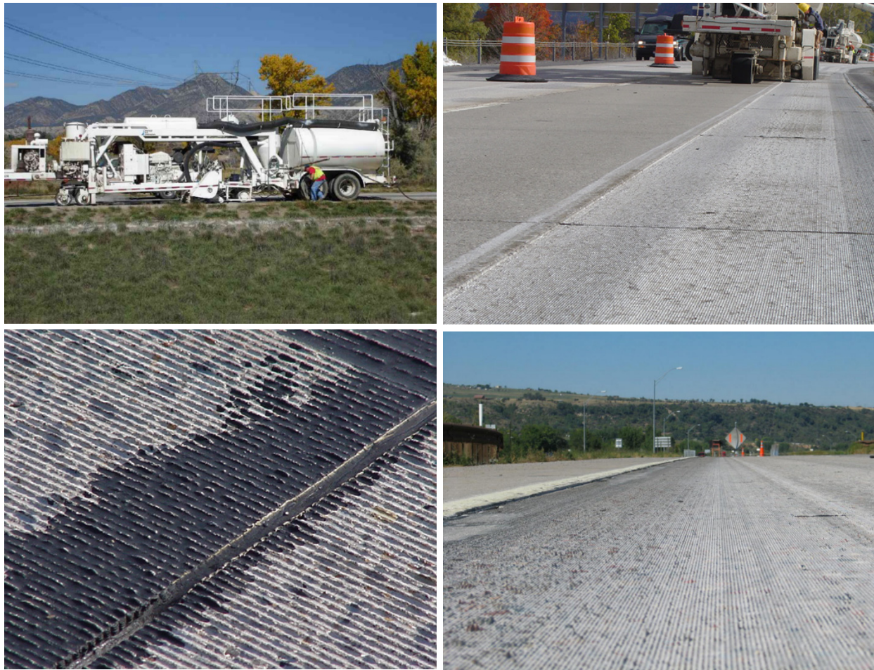
Figure 10-6. 2005 diamond grinding work (Necessary and Lemasany 2006).
