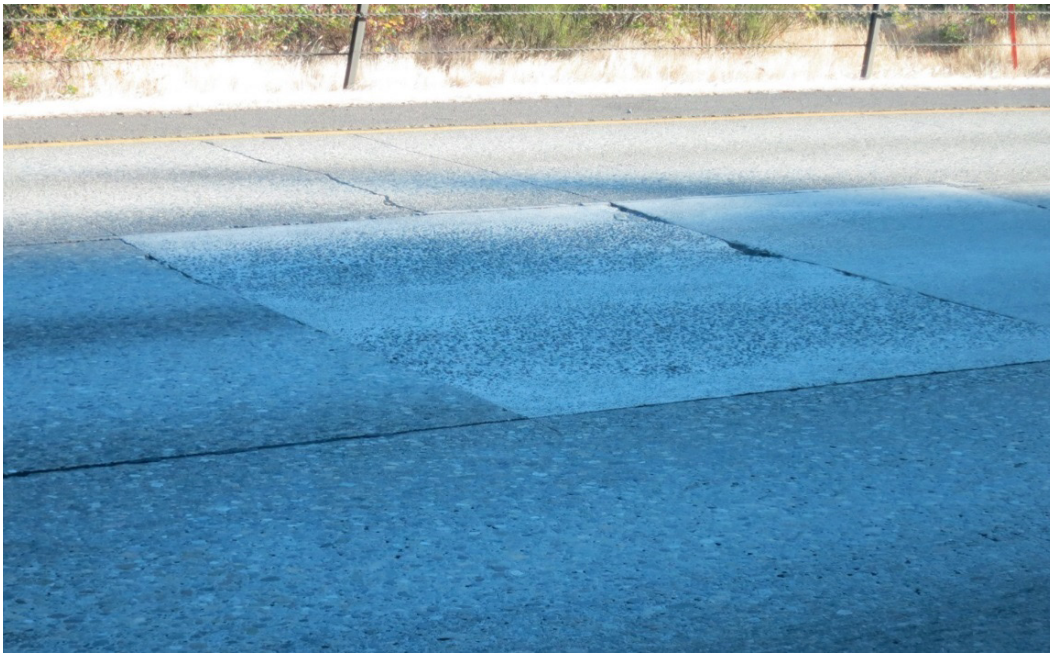
Figure 12-6. Replaced slabs showing signs of severe surface wear from studded tires.
