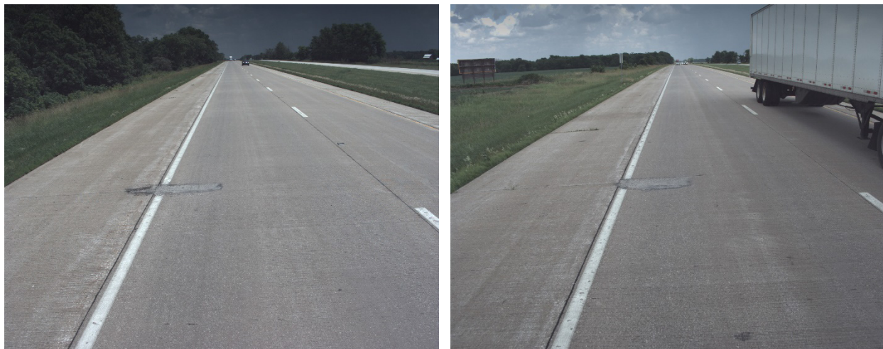
Figure 4-9. Punchouts between shoulder and driving lane addressed with temporary patching.
