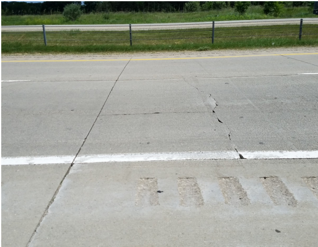
Figure 3-13. Isolated slab cracking linked to poor drainage.
