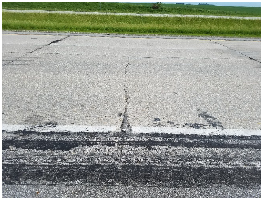
Figure 8-14. Example of mid-panel transverse cracking on U.S. 20 EB in 2018.
