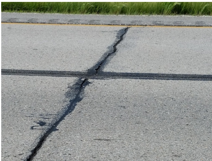
Figure 8-11. Typical transverse joint reflective cracking on U.S. 20 WB in 2018.
