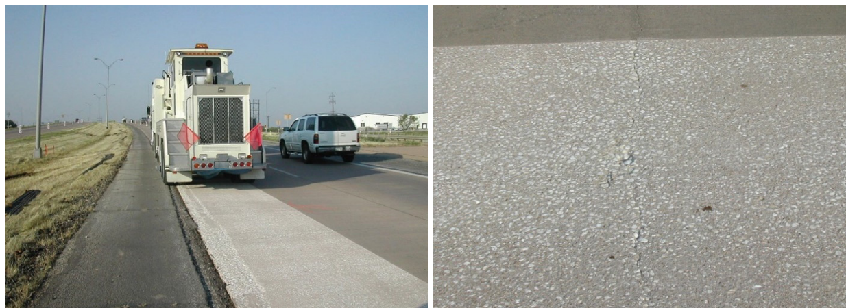
Figure 7-3. Shotblasting operation (left) and resulting surface texture (right) (Won 2016).
