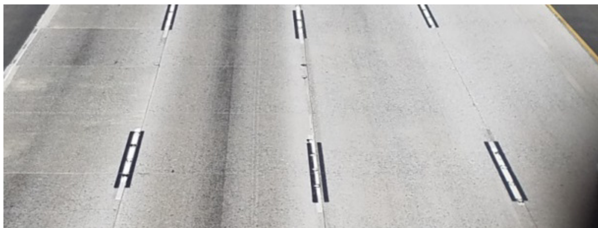
Figure 11-3. View (towards oncoming traffic) of the existing concrete pavement in 2018. Left two lanes are original concrete pavement.
