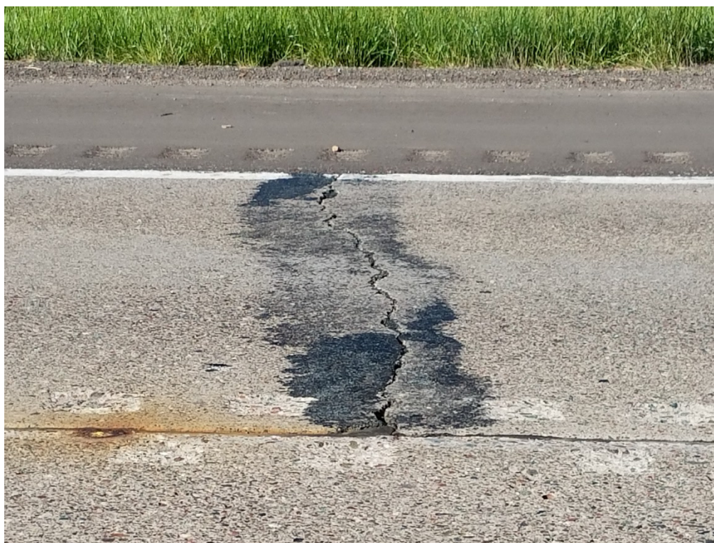
Figure 9-6. Medium-severity mid-panel crack with temporary asphalt “repair.”
