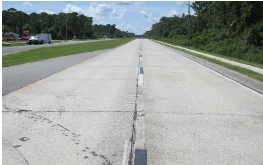
Figure 6-3. Overview of concrete overlay, SB U.S. 1 in 2018.
