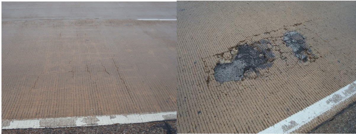
Figure 7-15. Areas of overlay deterioration, possibly indicating localized loss of bond.
