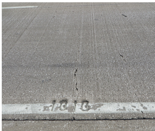
Figure 4-7. Spalling along transverse crack (left) and punchout (right).
