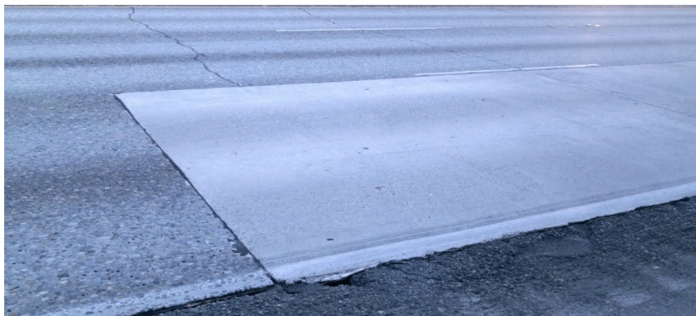
Figure 12-5. Slab replacement in outer (truck) lane and medium-severity transverse crack in center and inner lanes.
