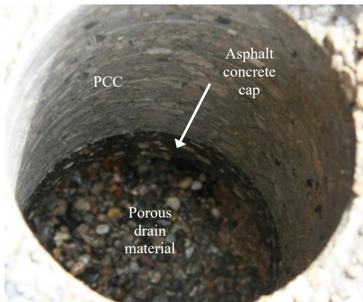
Figure 3-11. Example of asphalt concrete cap over edge drain.
