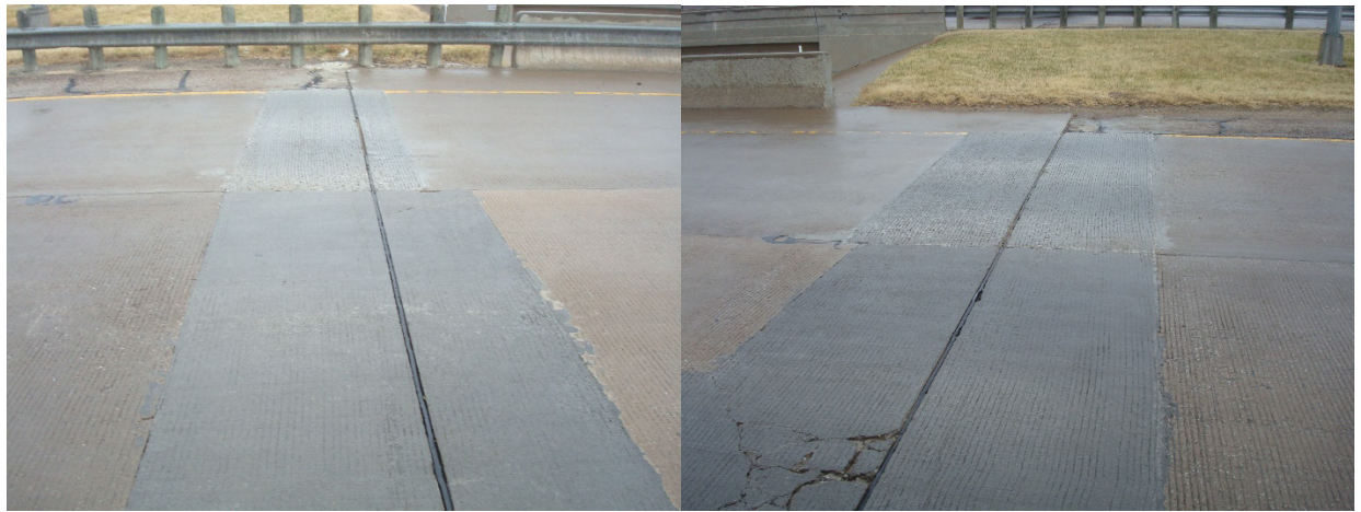
Figure 7-12. Typical 2016 patching at bridge approach transitions.
