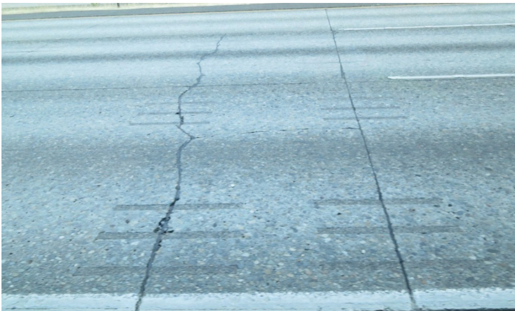
Figure 12-7. Dowel bar retrofit across transverse joint and crack.
