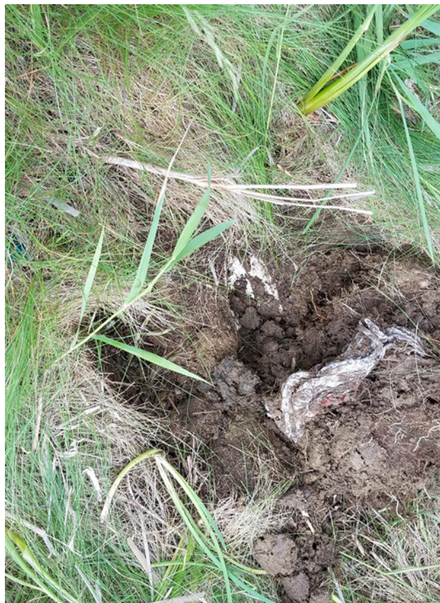
Figure 3-11. Example of asphalt concrete cap over edge drain.
