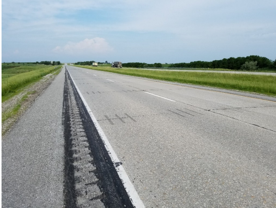
Figure 8-12. Overview of U.S. 20 EB with DBR and diamond grinding in 2018.
