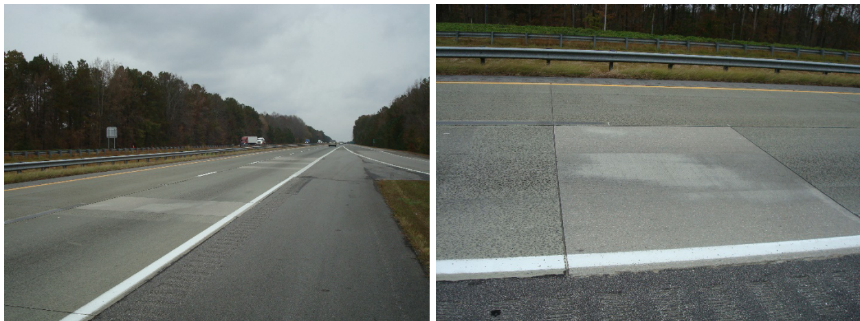
Figure 5-10. Examples of full-depth repairs near rest area (~MP 198.5) on NC I-85 overlay project.
