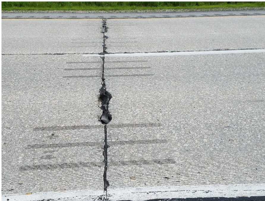
Figure 8-13. Example of spalling and joint seal damage on U.S. 20 EB in 2018.
