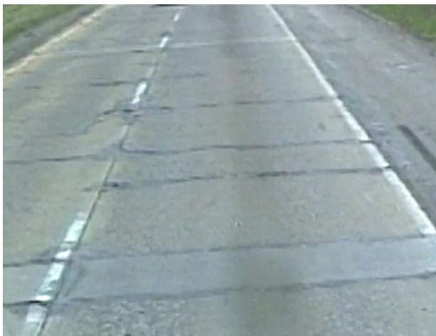
Figure 3-2. Typical condition of JRCP prior to UBOL.
