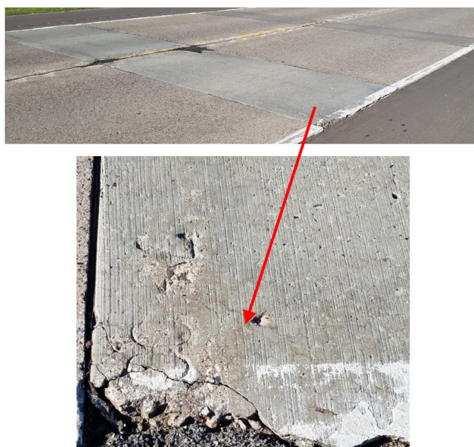
Figure 9-11. Example of 2000 repair condition in 2018 showing map cracking and corner spalling.
