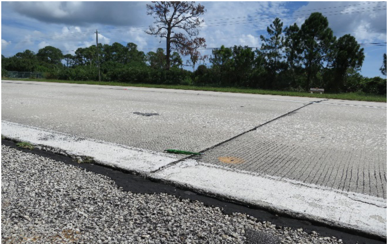
Figure 6-5. Minor faulting on 7-inch slab with special dowel configuration in 2018.
