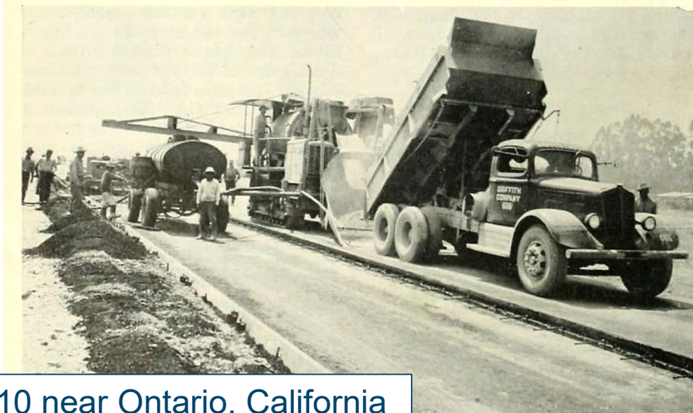
Concrete paving on bituminous treated subgrade on the Ontario-to-Colton Freeway
