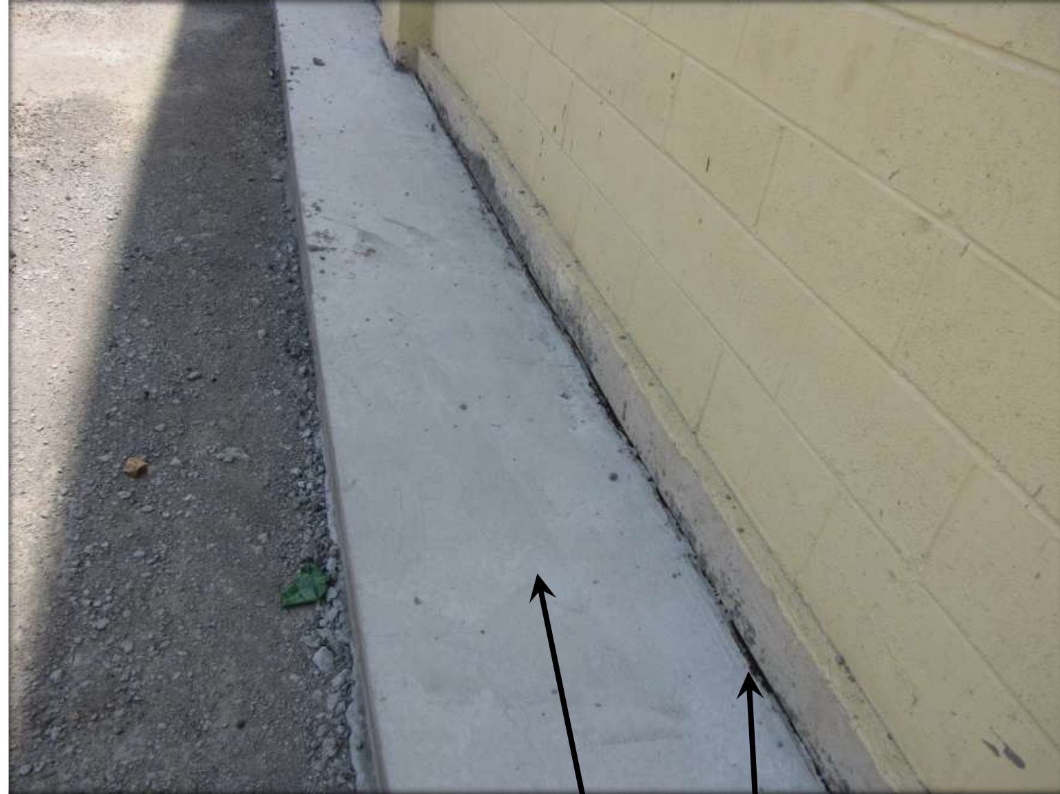
PCC Apron at building wall
