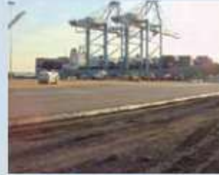
Late 1980s–early 1990s: RCC pavements are constructed for automotive, port, and intermodal facilities in the U.S.
