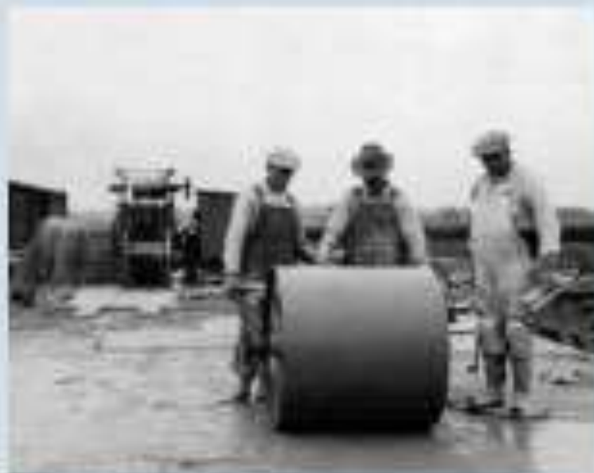
Early 1940s: The first RCC pavement in North America is an airport runway constructed in Yakima, Washington.
