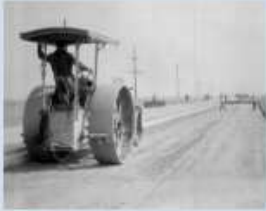
1930s: A form of RCC paving is performed in Sweden.
