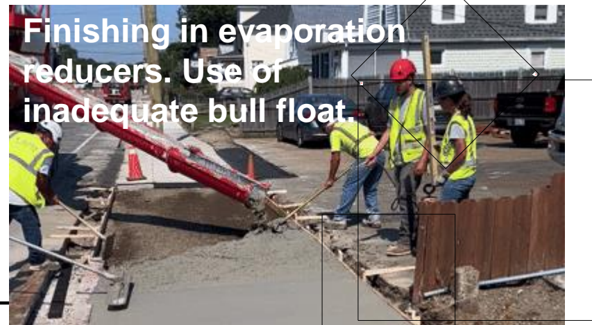
Pushing broom. Use of walking floats.
