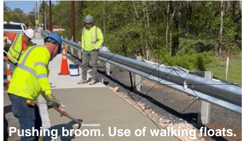
Finishing in evaporation reducers. Use of inadequate bull float.
