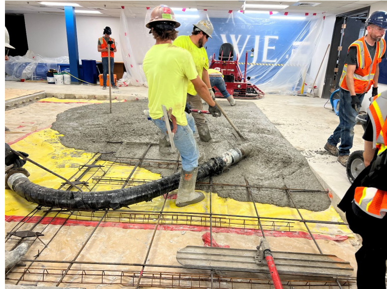
Pumping Concrete
