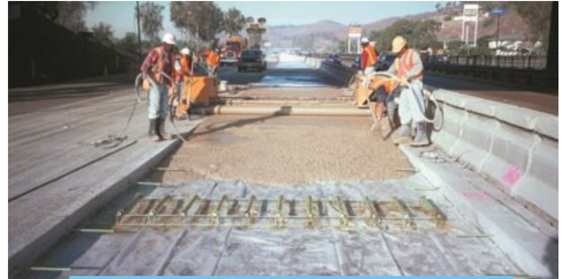
Construction of JPCP-RSC on I-10 in 1999
