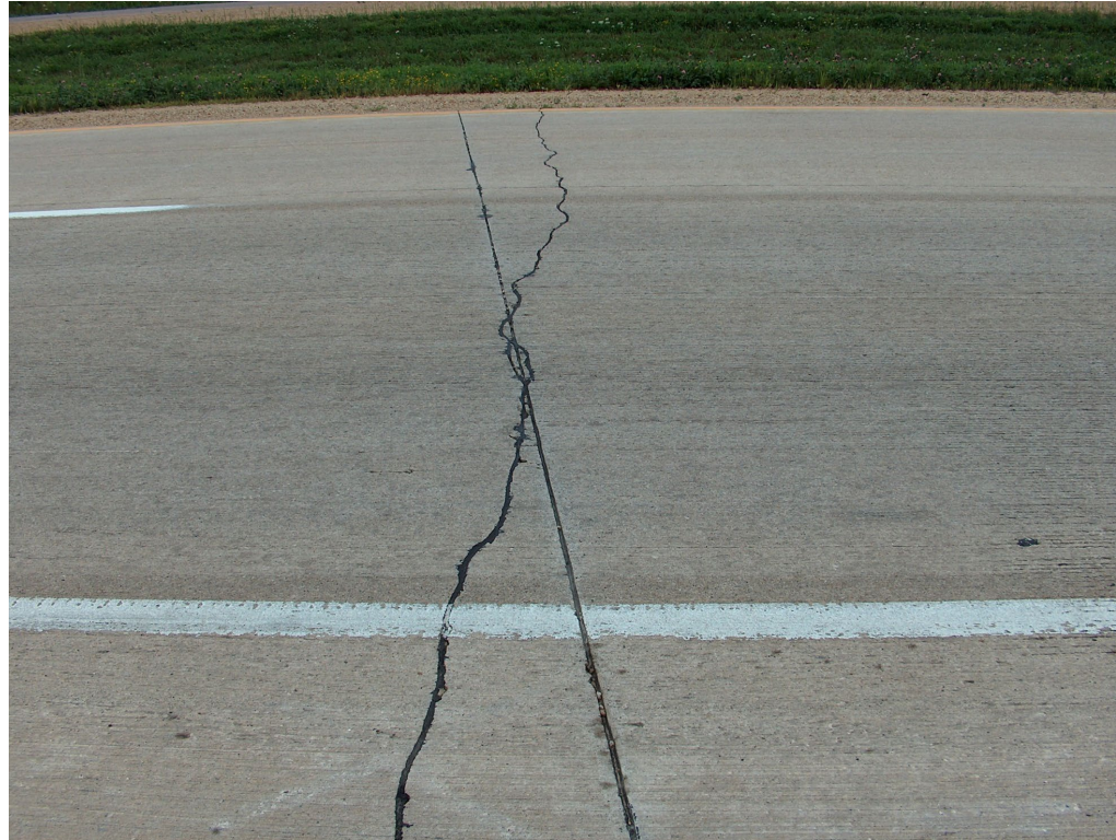
Late sawing crack
