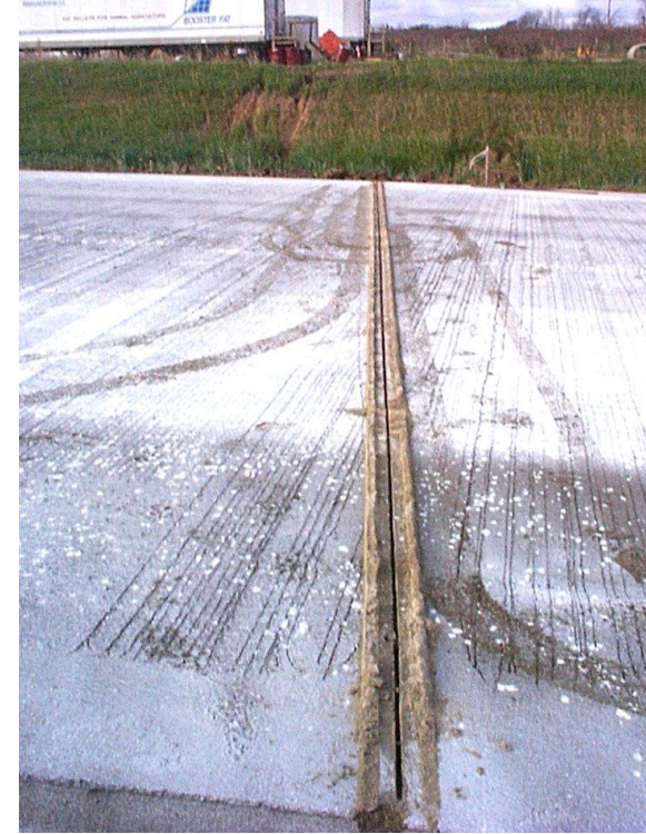
Residue from early entry sawing
