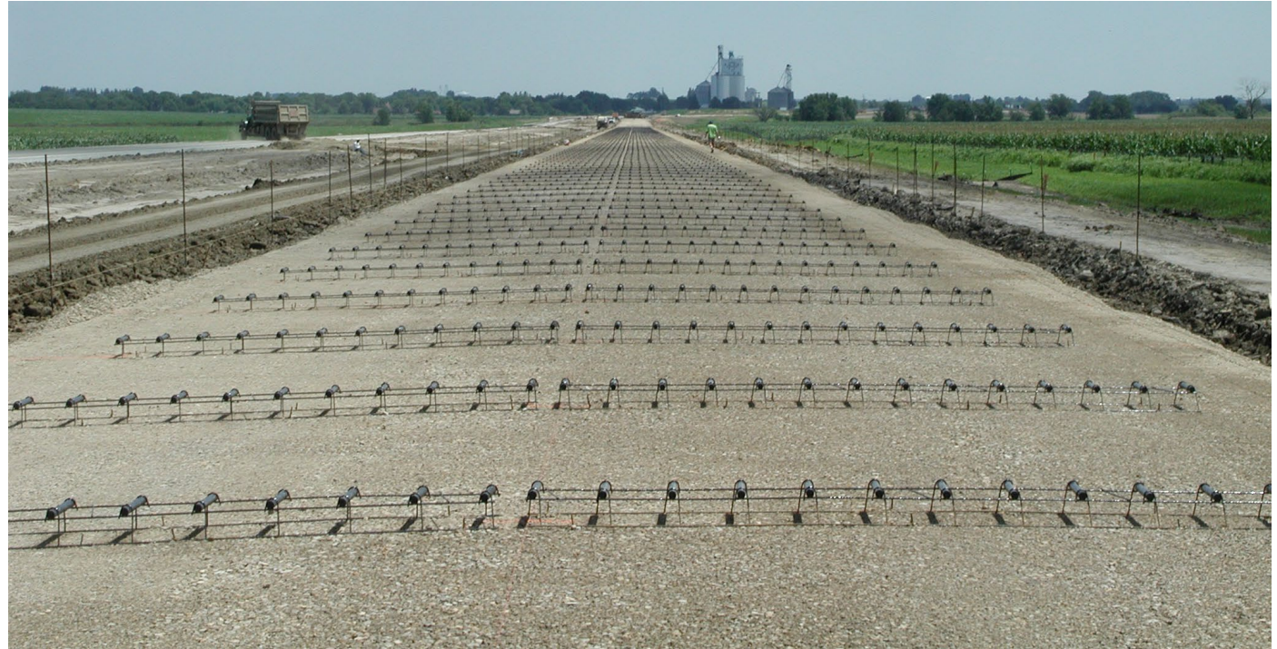
Sighting the grade for dowel alignment
