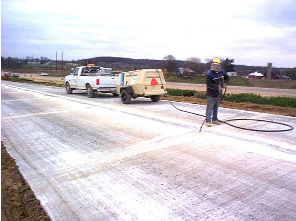
Air blast of joint prior to sealing
