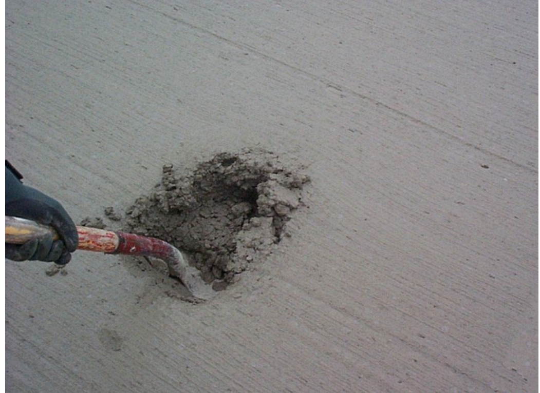
Sampling concrete behind the paver
