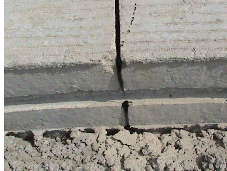
Blowout at edge of slab
