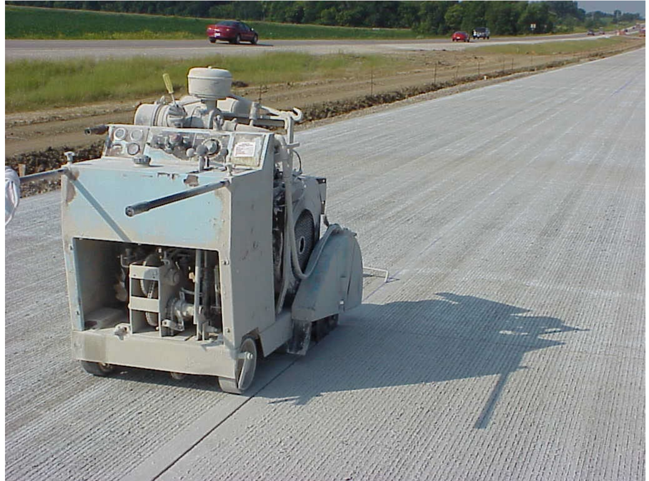
Conventional saw on longitudinal joint
