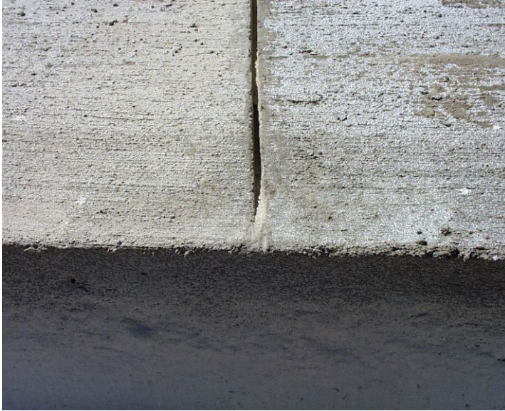
Pull up of sawcut before edge of slab
