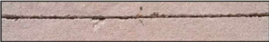
b) Moderate raveling—sawed early in the window
