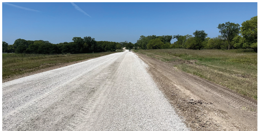
Aggressively rehabilitated and chemically stabilized gravel road
