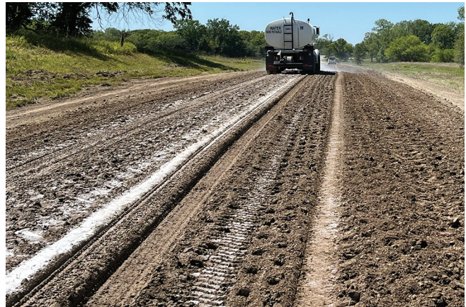
Stabilizer being sprayed onto subgrade
