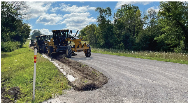
Excavation of ditch material
