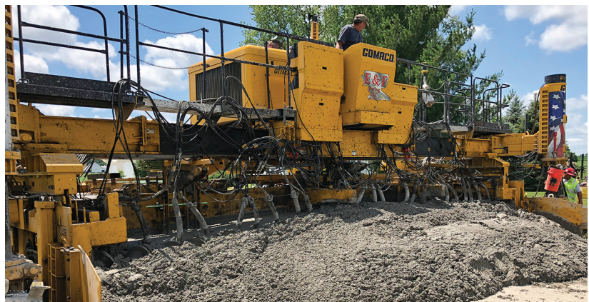
Washington County Road W-61 overlay placement
