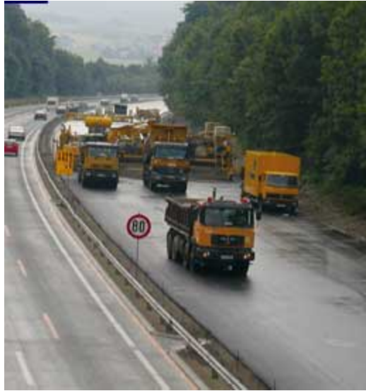
Figure 1. Two-lift paving in Austria
