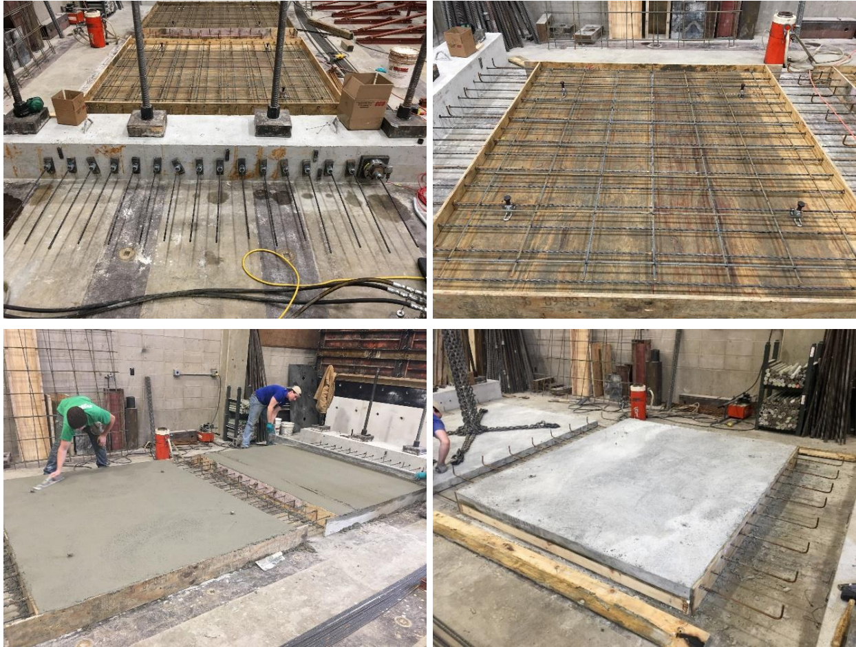
Figure 13. Construction of precast prestressed interior deck panel
