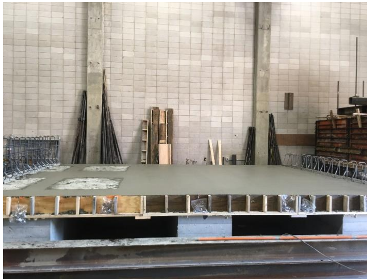
Figure 18. Construction of CIP concrete and barrier
