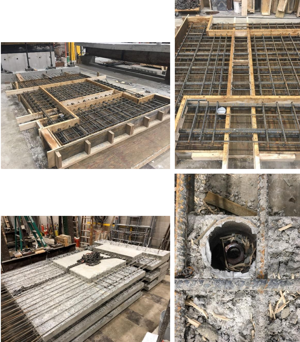
Figure 14. Construction of precast double-panel overhang (exterior panel)
