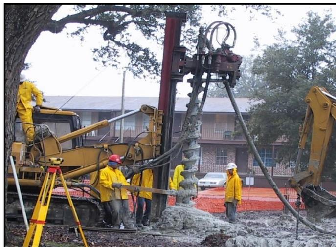
**Figure 2-7. Equipment used for low headroom continuous flight auger piles**
