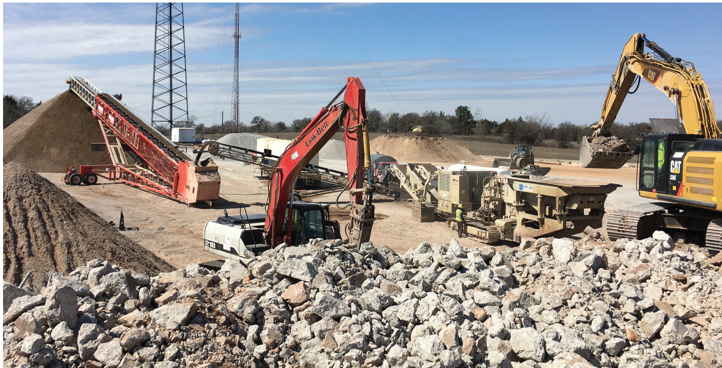
Figure 5. Typical concrete pavement crushing and stockpiling operation
