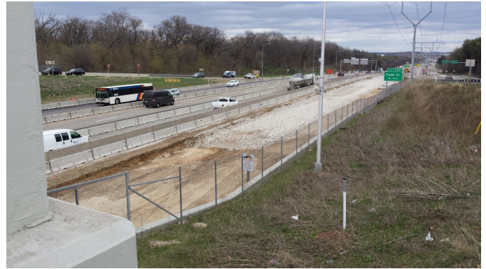
Figure 4. RCA spread for base course (Photo courtesy of Eleanor Bloom, Recycled Materials Resource Center)
