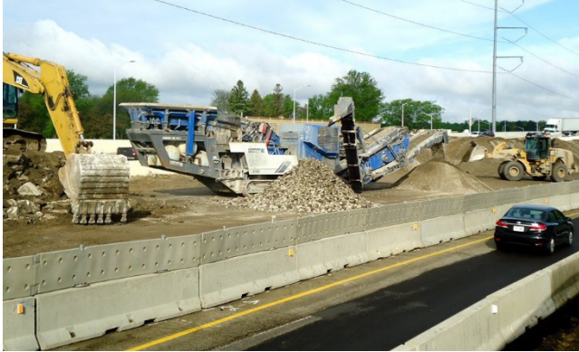
Figure 3. Onsite crushing operations at the Beltline Highway project (Photo courtesy of Steven Theisen, WisDOT)
