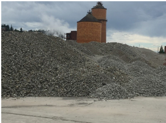
Figure 7. RCA produced and stockpiled off-site for James Street Bridge Replacement (Photo courtesy of Freeman Anthony, City of Bellingham)
