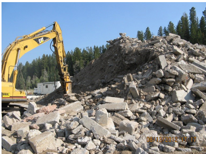
Figure 5. Pile of waste concrete prior to crushing into RCA (Photo courtesy of Phillip Lamoureux, FHWA WFL)
