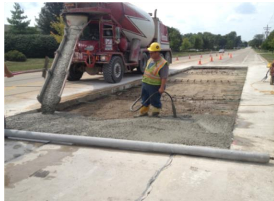
Figure 5. Example of internally cured concrete being used for concrete pavement patching
