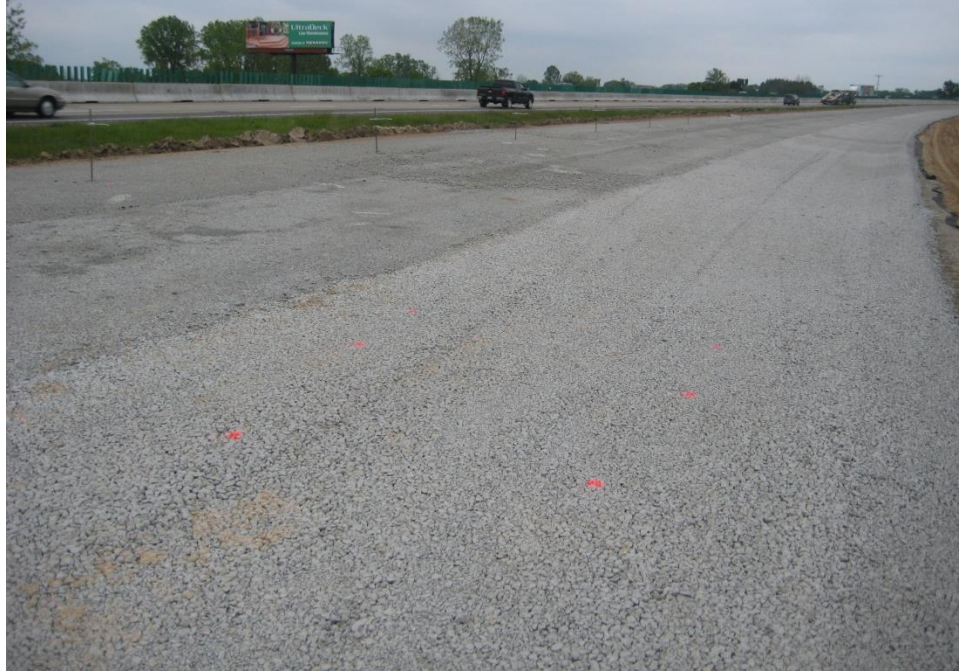
Figure 11. MI I-96 TS2 CTB layer (looking east near Sta. 296+25)
