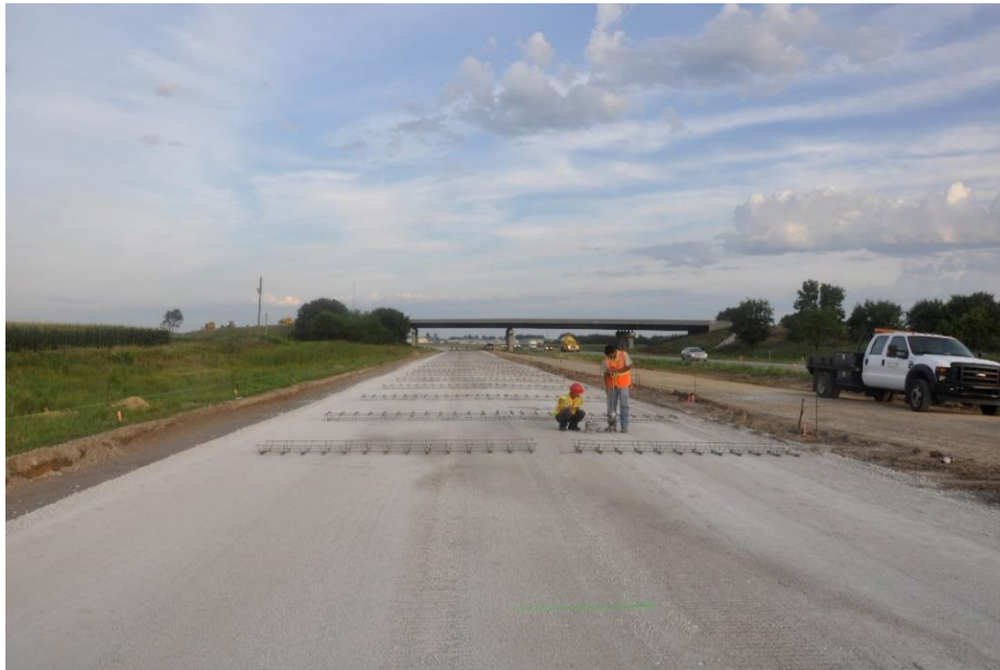
Figure 15. IA US30: Field testing on finished RPCC modified subbase layer (June 8, 2011)
