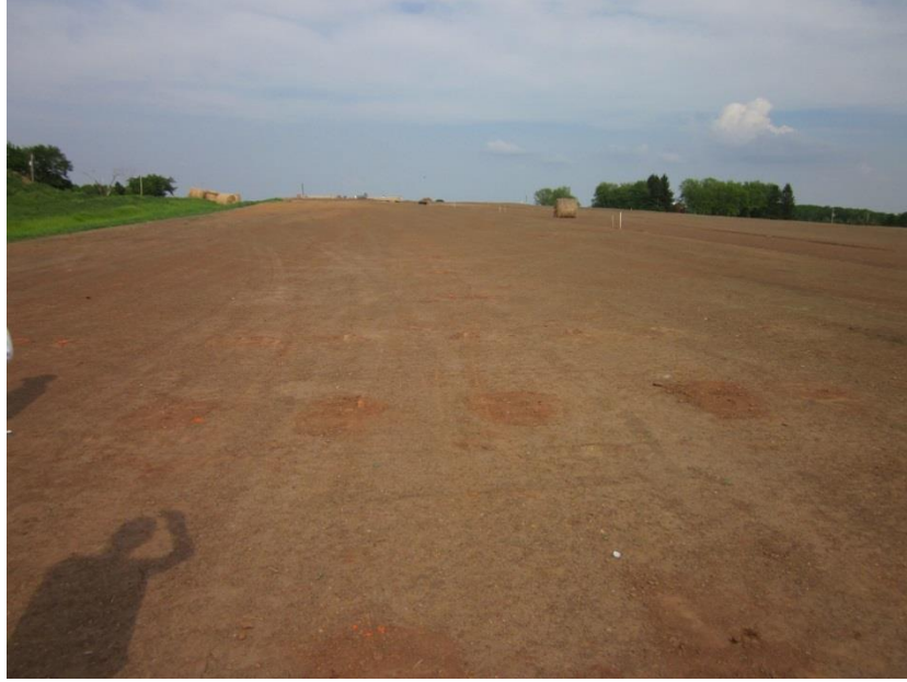
Figure 13. WI US10 TS2: Photograph of the compacted subgrade
