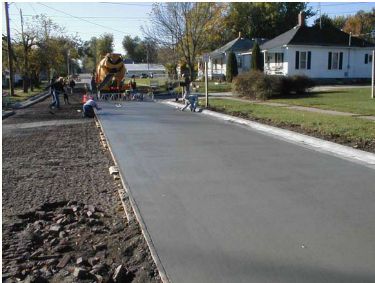
Figure 6. Southbound lane overlay paving
