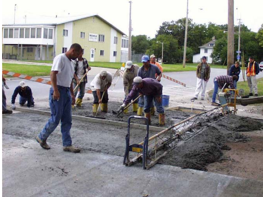
Figure 16. Initial concrete overlay placement
