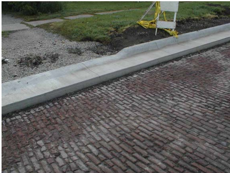
Figure 5. Finished curb and gutter unit
