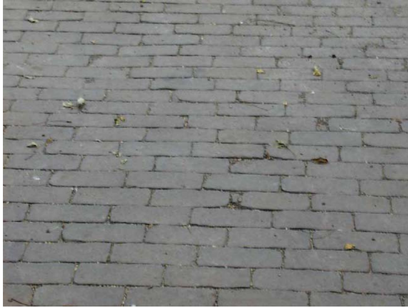
Figure 13. Air blasted surface
