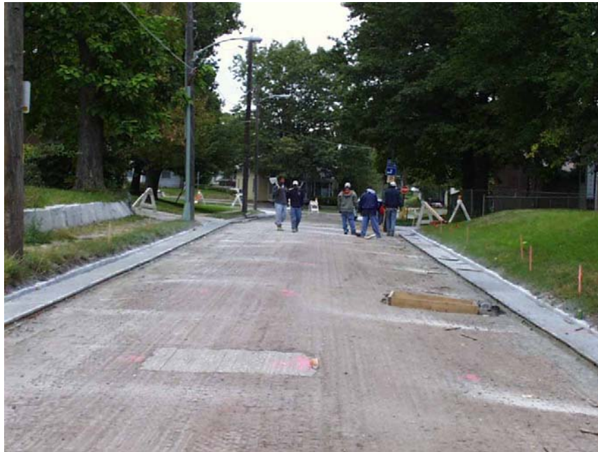
Figure 12. Replacement curb and gutter units in place
