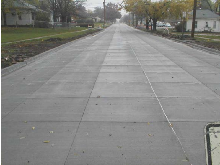
Figure 8. Completed jointing pattern
