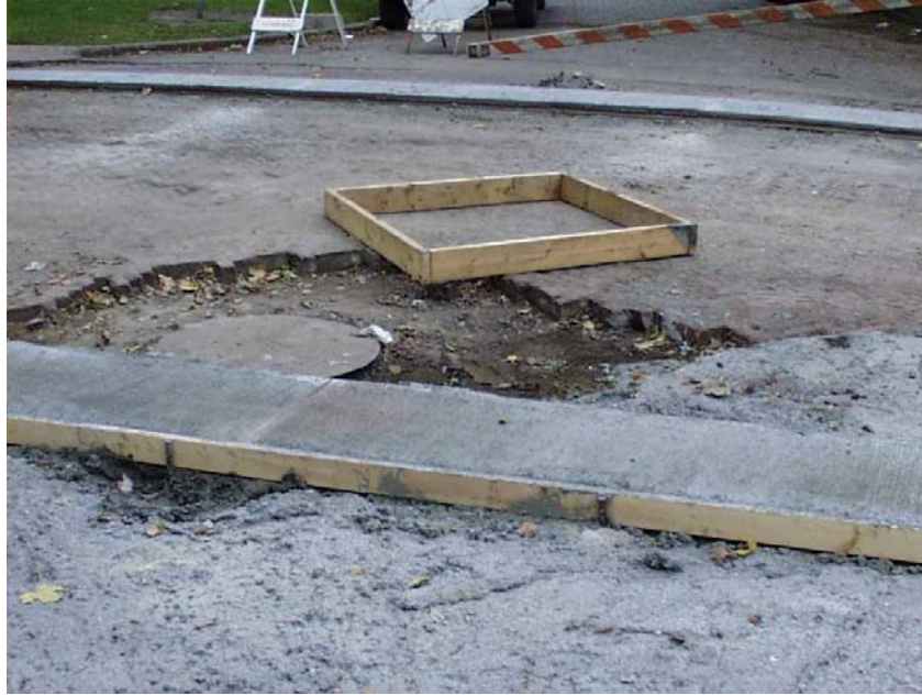
Figure 15. Manhole box out preparation
