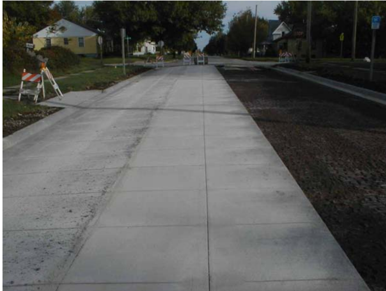
Figure 7. Southbound lane paving completed
