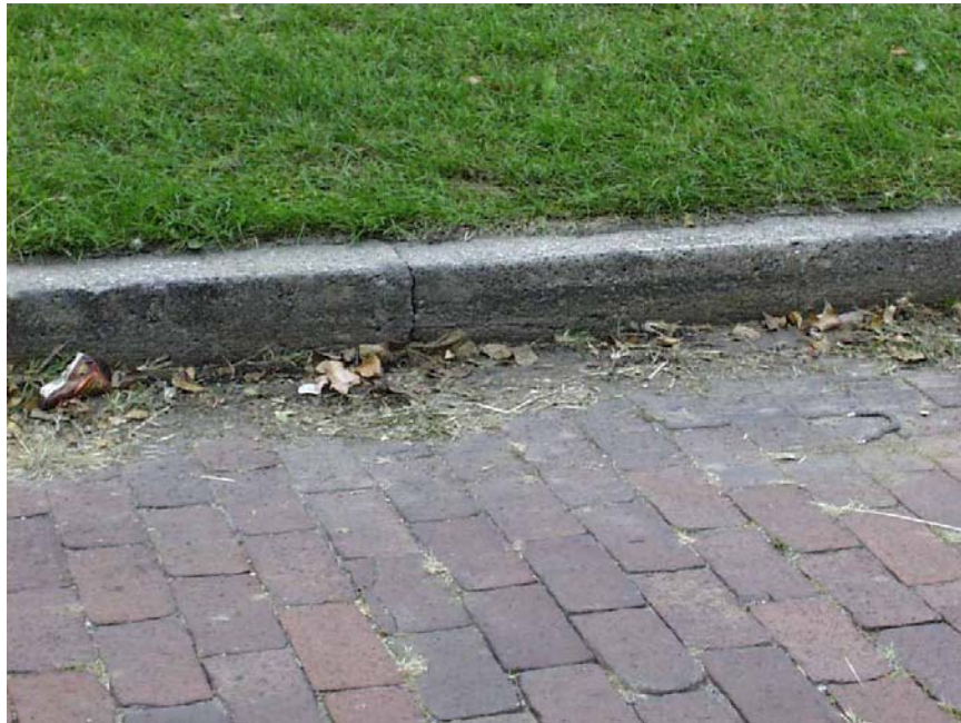
Figure 10. Existing pavement and bull-curb
