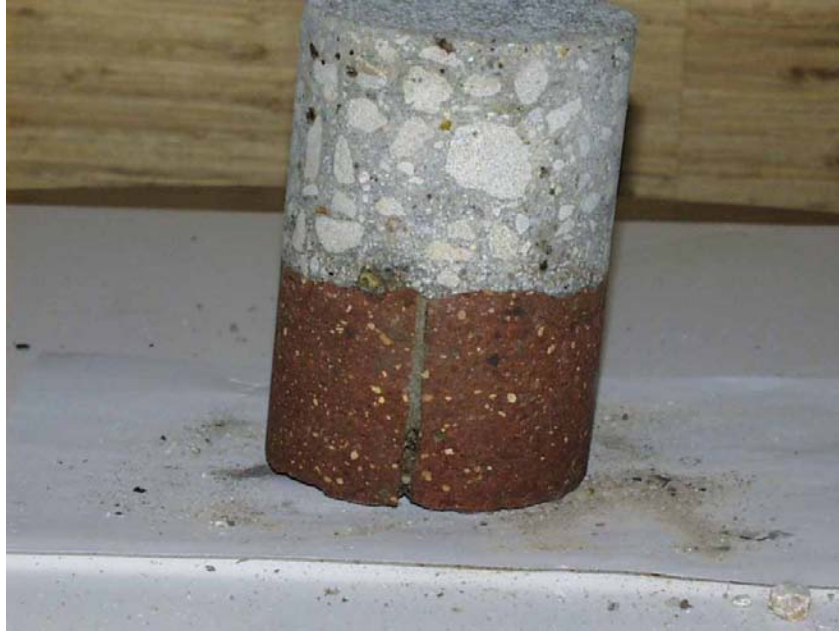
Figure 18. PCC over brick core
