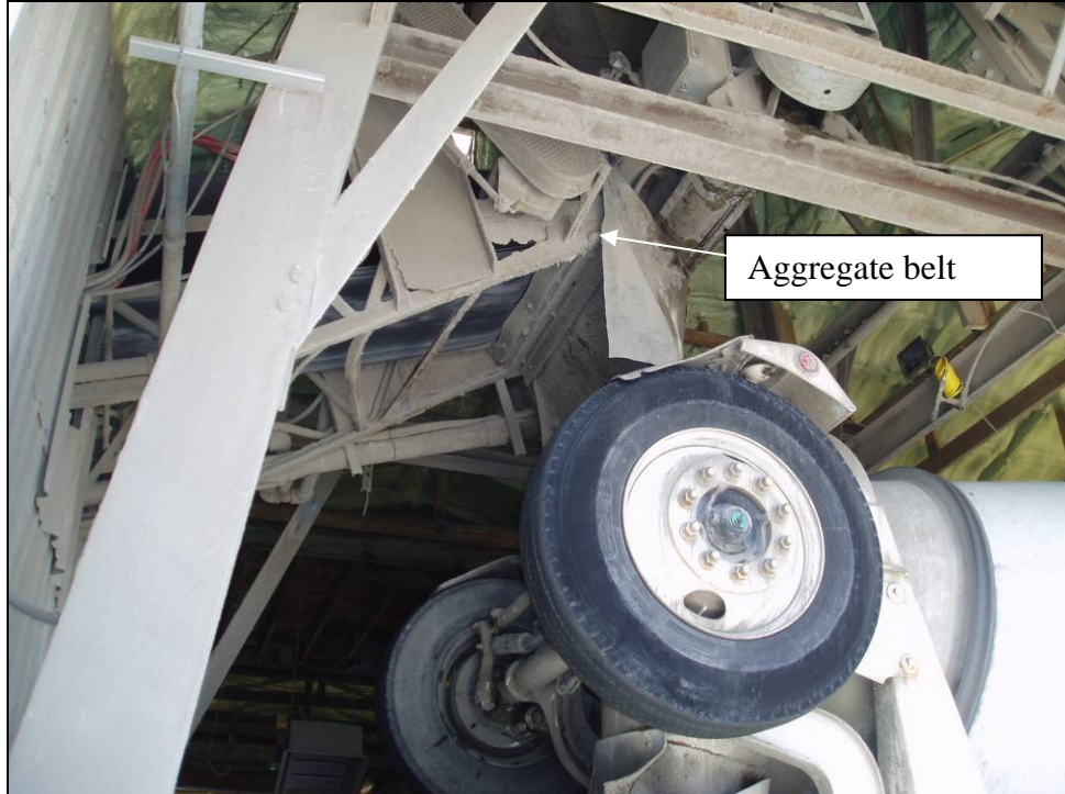
Figure 47. Aggregate belt charging ready mix concrete truck
