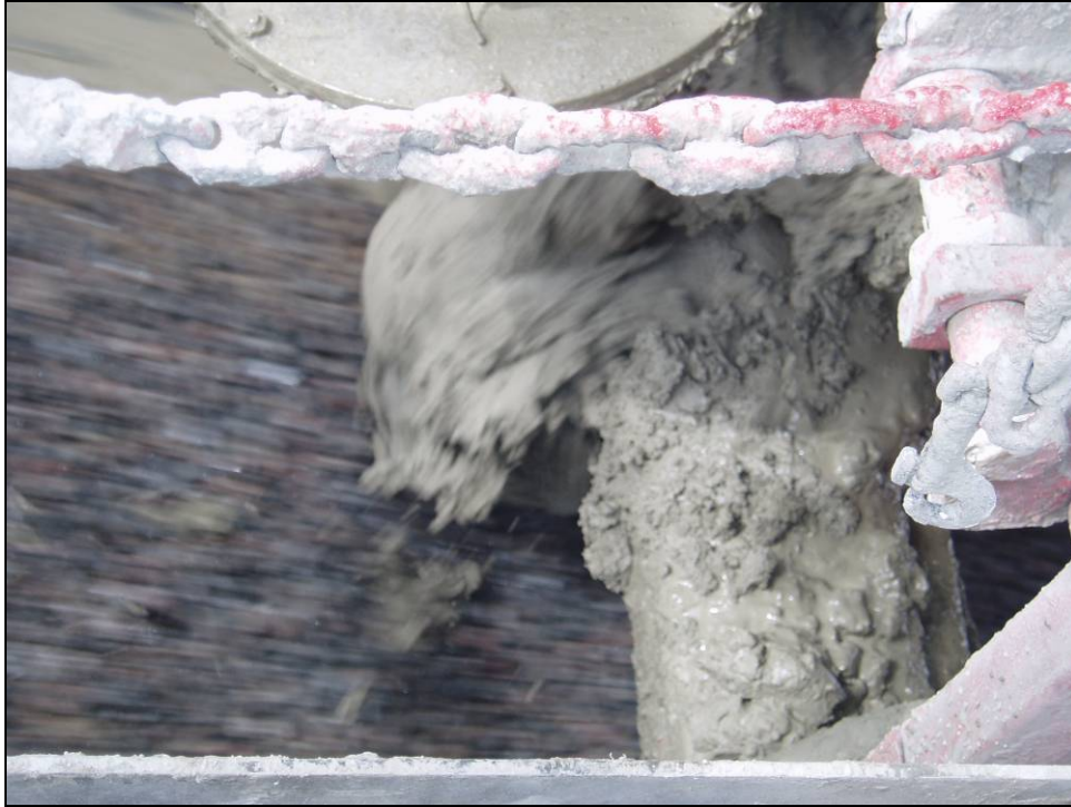
Figure 53. Slurry being charged with aggregate
