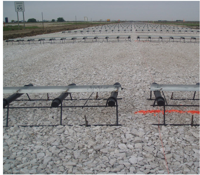
Cross-section of joint-forming device on top of the dowels
