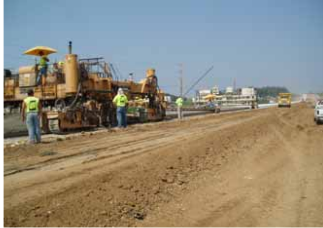
Figure 2. Paving train
