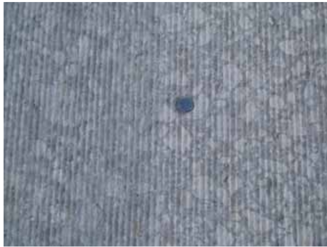
Figure C37. Diamond grinding
