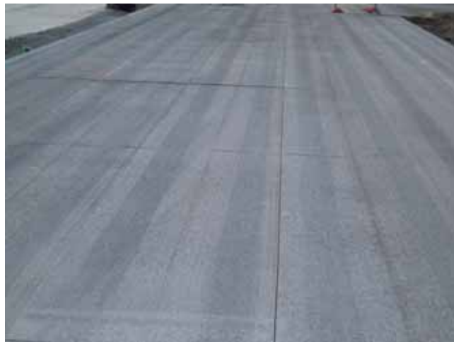
Figure C38. Diamond grinding
