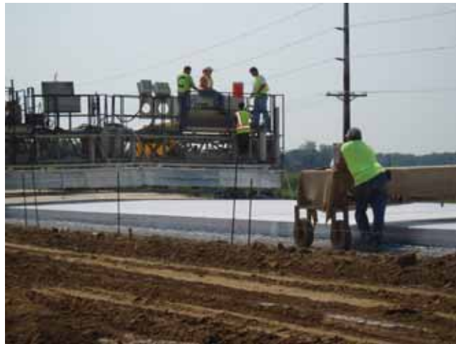
Figure 3. Tining machine operations
