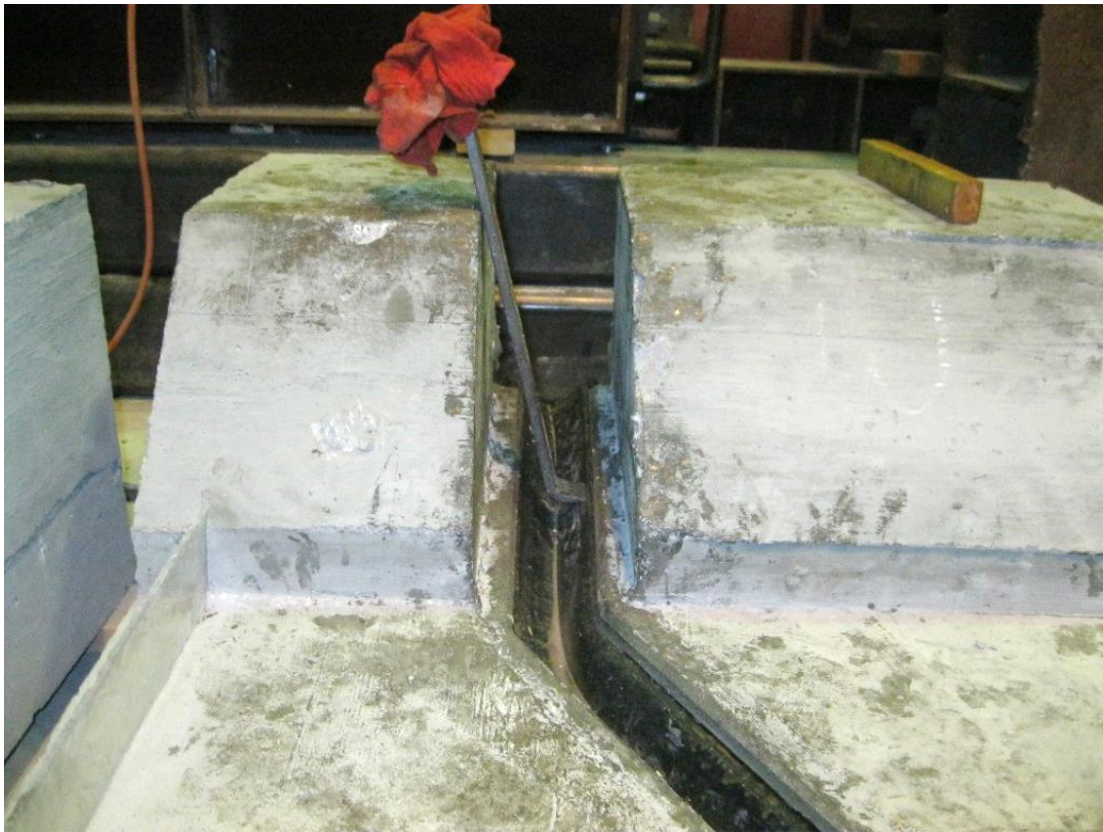
Figure 51. Watson Bowman Acme gland installation tool limited by mid-height barrier rail
