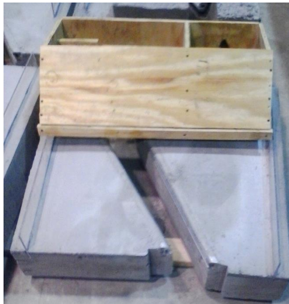
Figure 30. Barrier rail formwork
