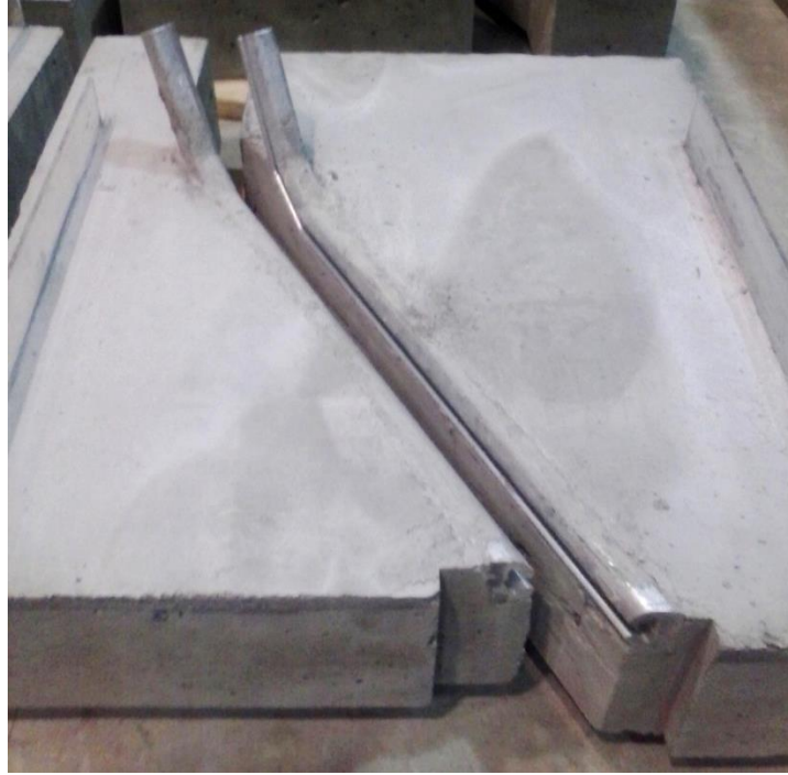
Figure 29. Strip seal construction before barrier rail placement
