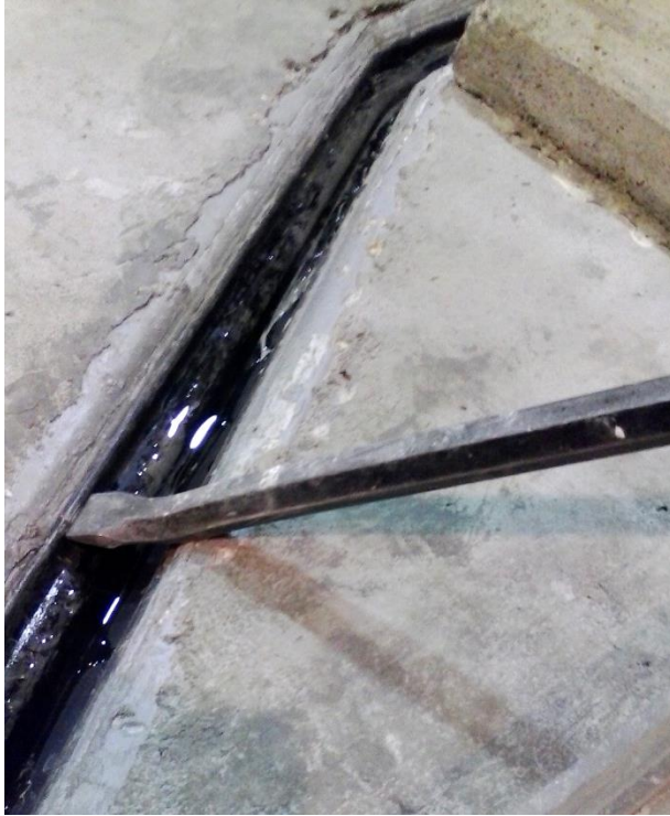
Figure 19. D.S. Brown gland installation
