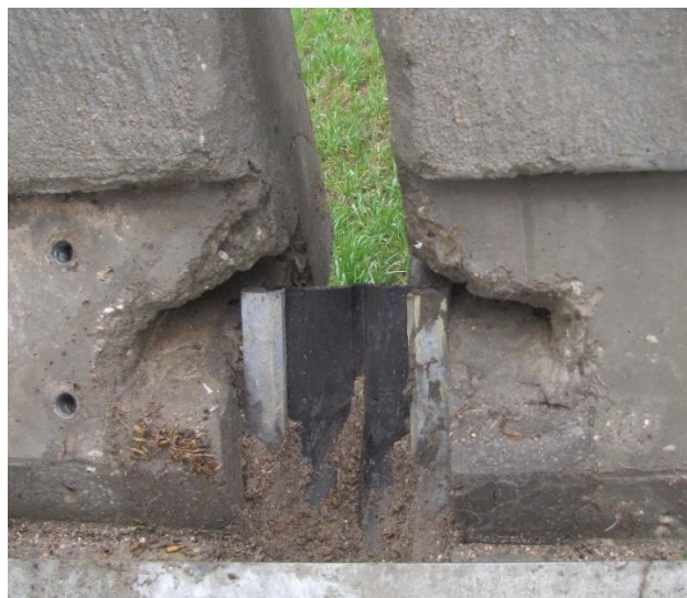
Figure 6. Finished construction of termination detail
