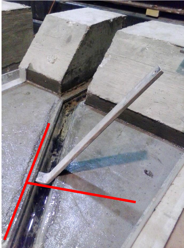
Figure 21. Watson Bowman Acme gland installation
