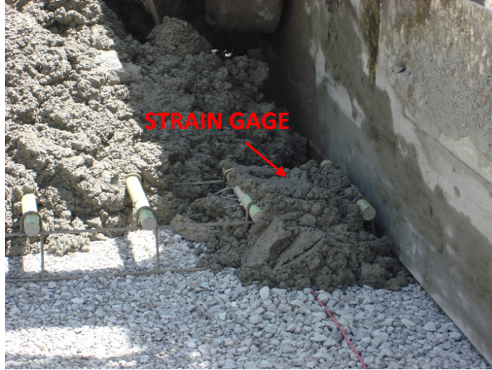
Figure 12. Strain gages during paving
