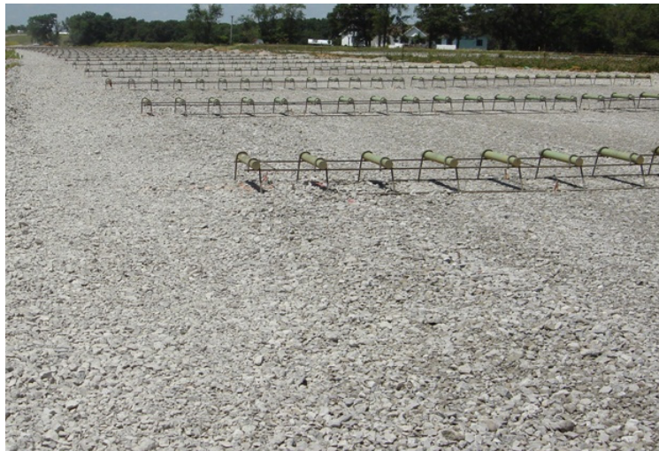
(b) Cables after installation
