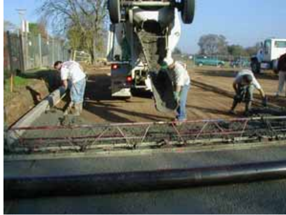
Figure 3. Vibratory screed used in placing PCPC
