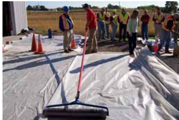
Figure 4. Transverse steel roller over the moisture barrier
