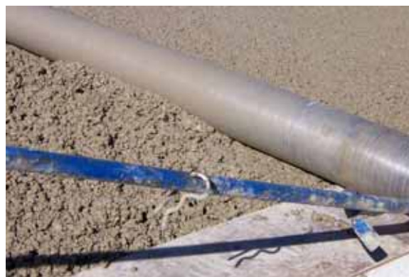
Figure 5. Compaction and finishing using a roller screed
