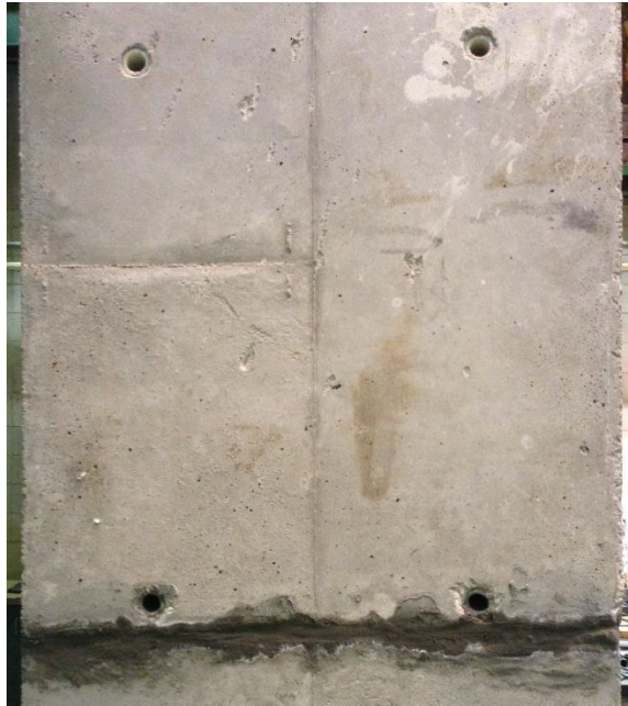
Figure 13. Port plugs before grouting
