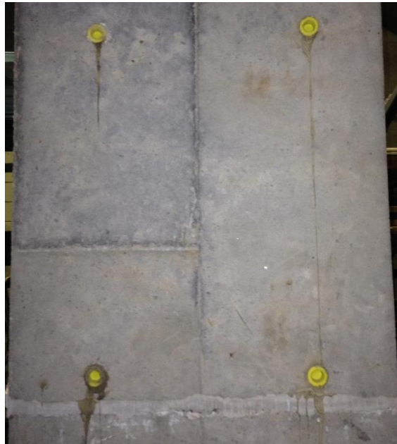
Figure 14. Port plugs installed after grouting
