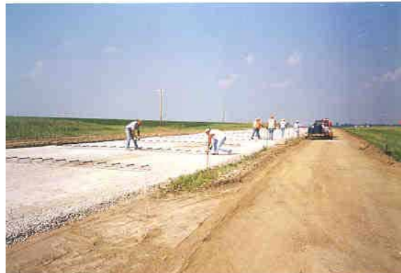
Figure 8. Placing baskets
