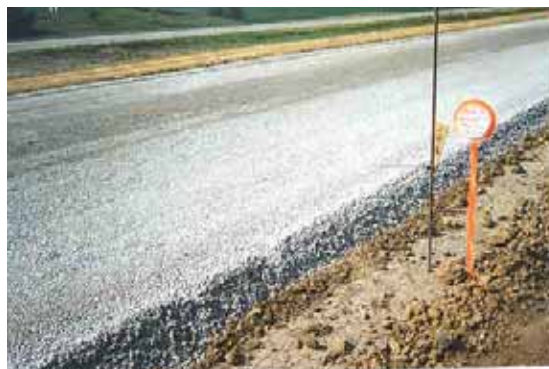
Figure 11. Marker at beginning of test site
