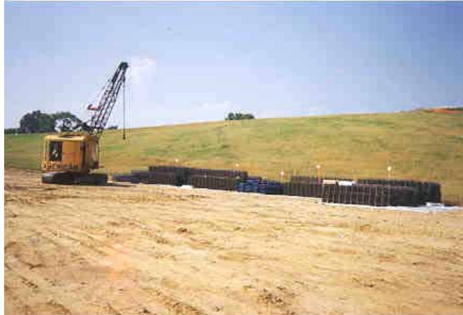
Figure 4. Staging yard with delivered baskets
