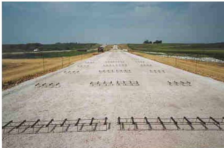
Figure 13. Baskets placed at wheel paths
