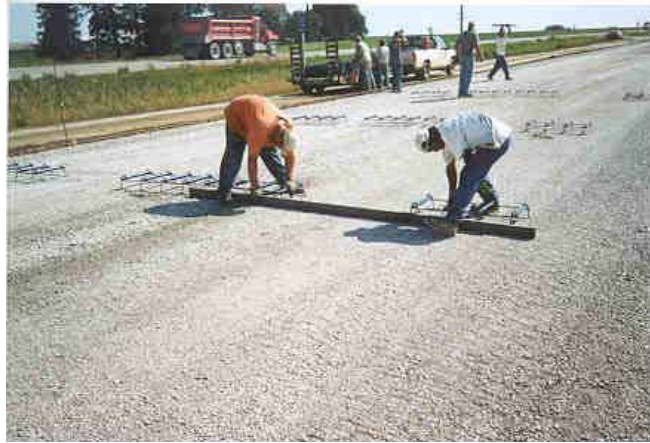
Figure 10. Setting baskets using aluminum jig
