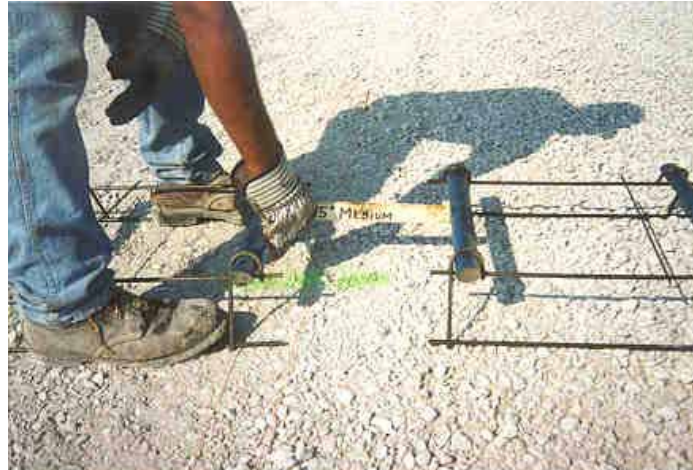
Figure 7. Spacing between baskets
