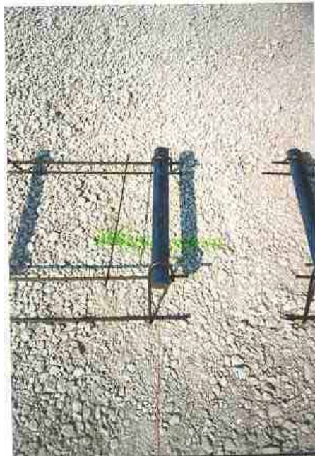
Figure 6. Inner dowel bar over offset line
