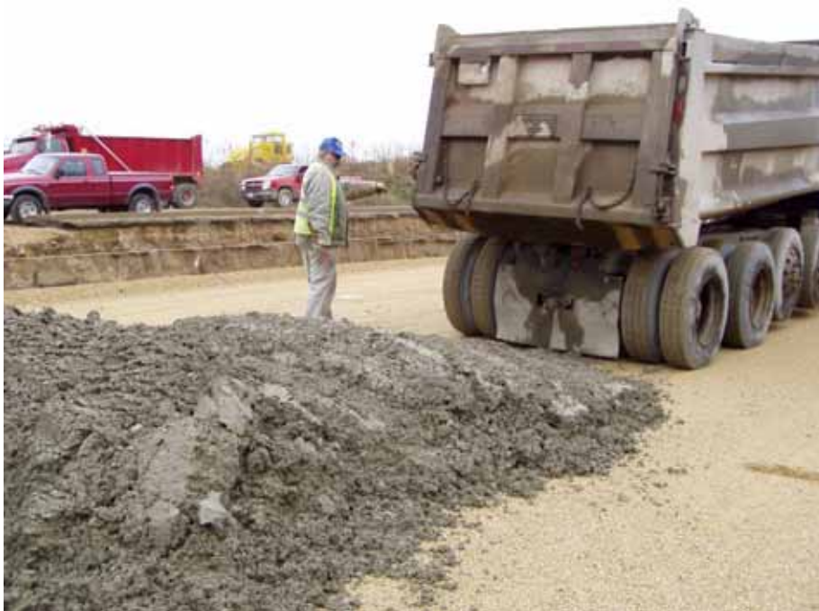
Figure A2. Concrete delivery operations
