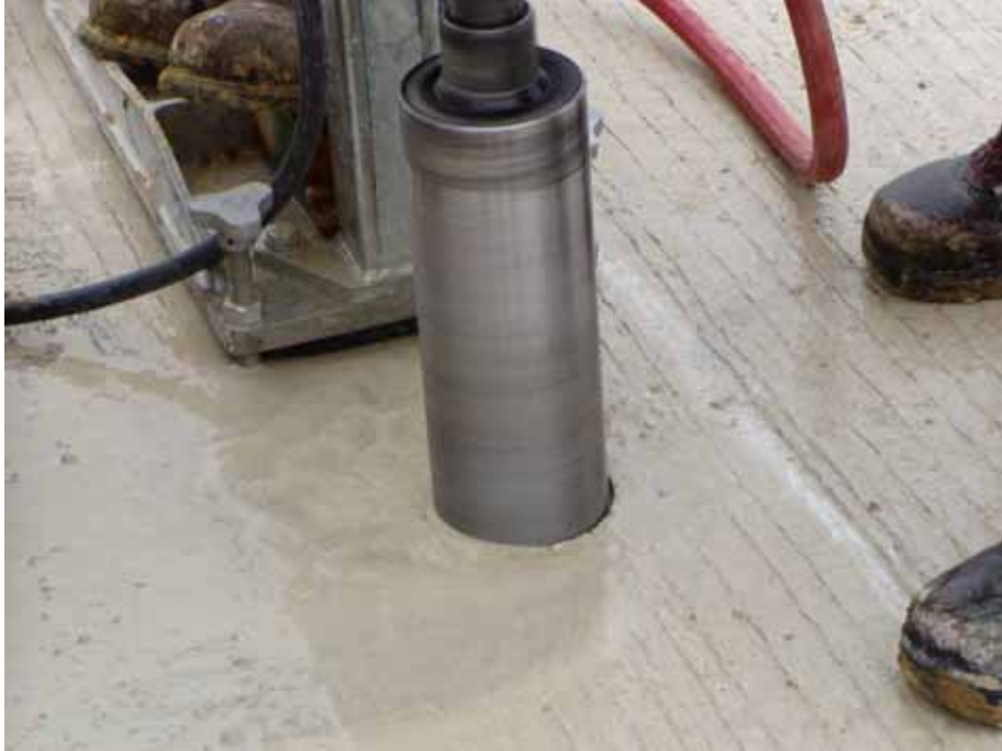
Figure A21. Pavement coring
