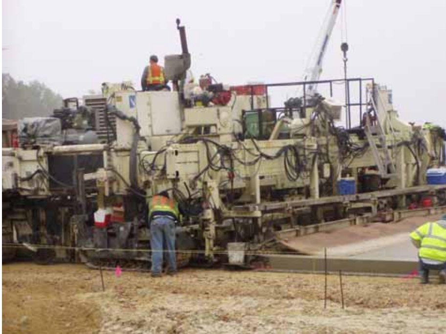
Figure A5. Paving operations
