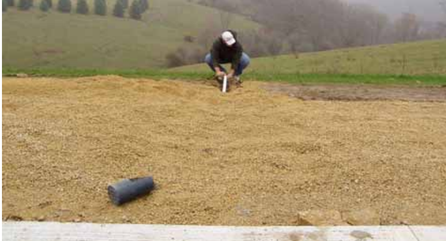
Figure 8. Temperature instrumentation leadwire protection for future access
