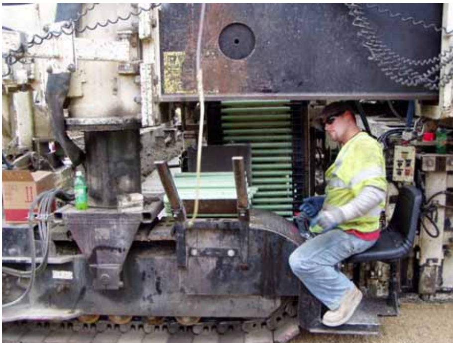
Figure A4. Dowel bar inserter operations
