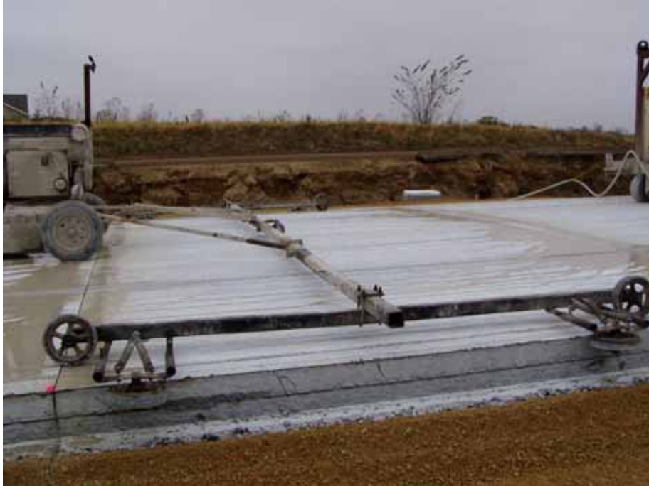
Figure A11. Longitudinal sawcut operations
