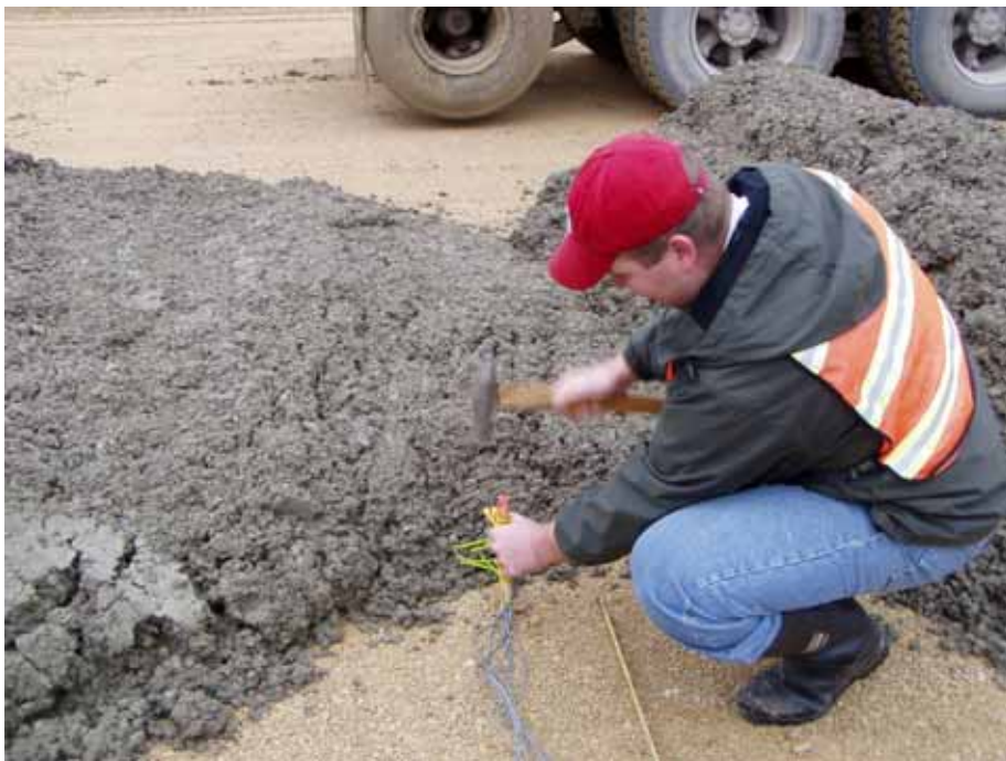
Figure A14. Temperature instrumentation installation
