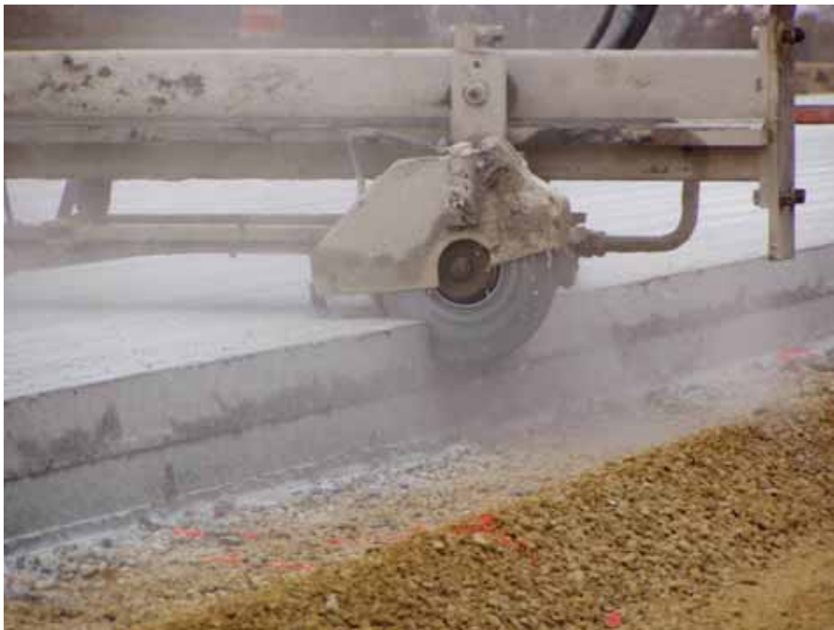
Figure A10. Transverse sawcut operations
