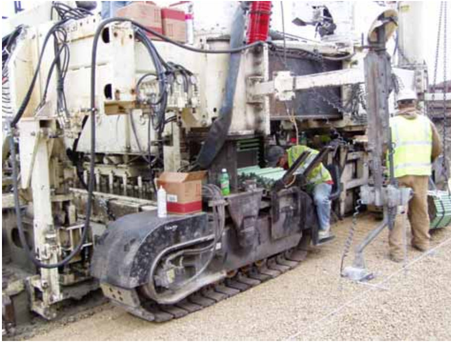
Figure A3. Paver and dowel bar inserter operations
