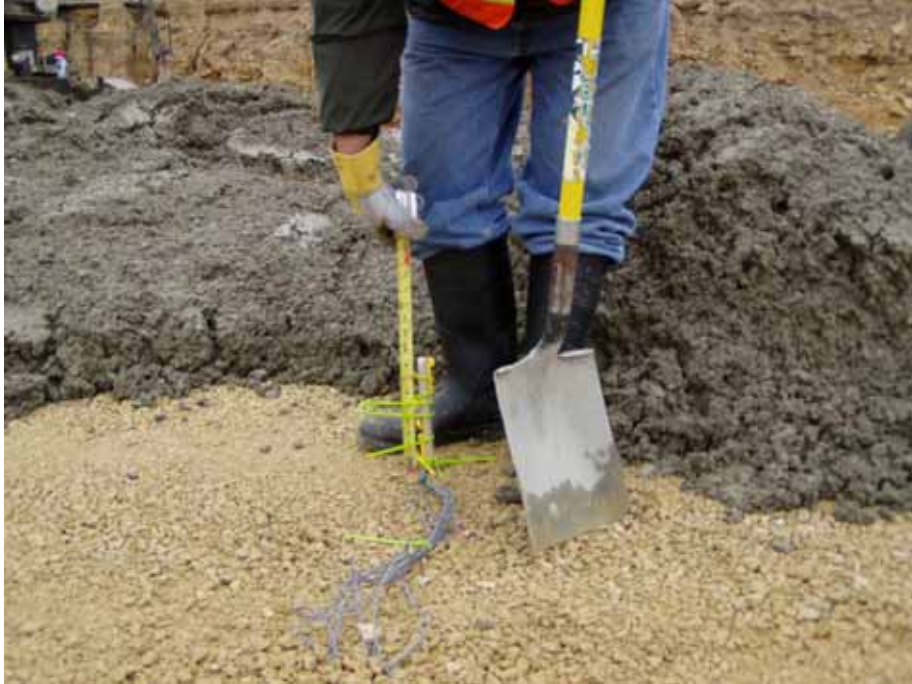
Figure A15. Temperature instrumentation installation
