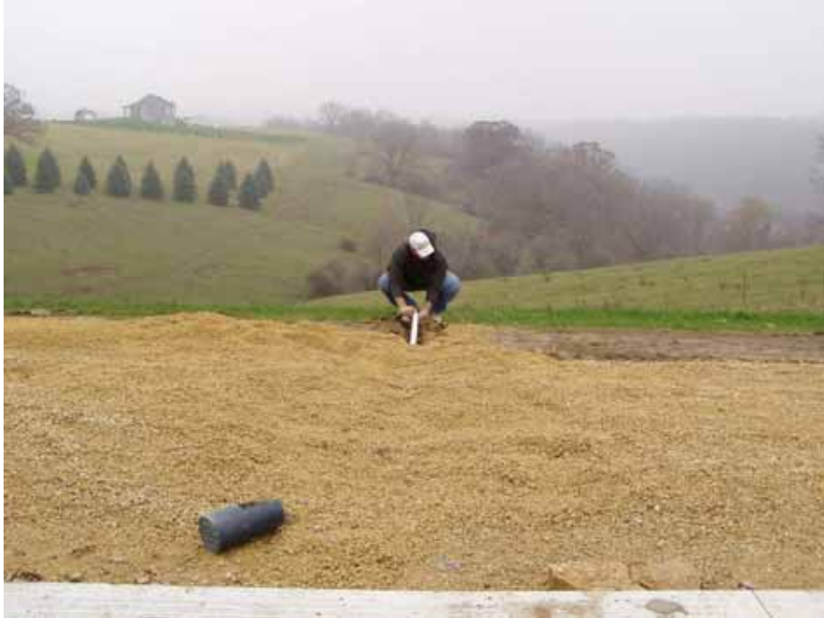
Figure A17. Temperature instrumentation installation
