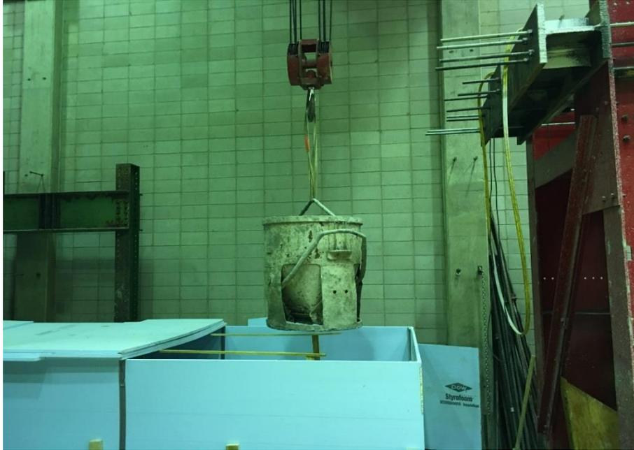
**Figure 30. Pouring joint concrete**
