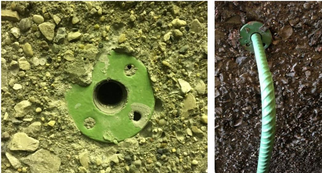
**Figure 18. Coupler embedded in the box girder concrete (left) and hook bar installed (right)**
