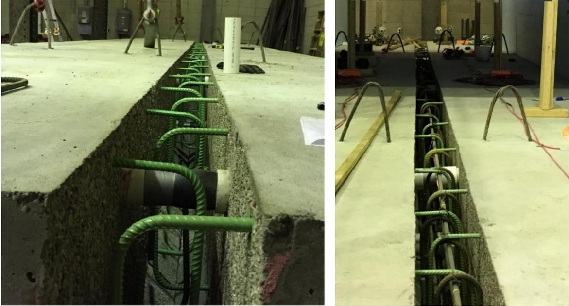
Two box beams placed side-by-side (left); Joint reinforcement with longitudinal bars and stirrups (right)
