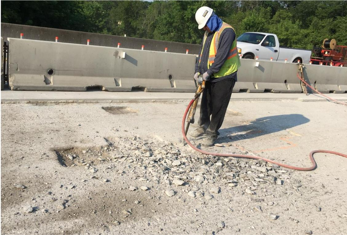
**Figure 4. Removal of unsound concrete using jackhammer**
