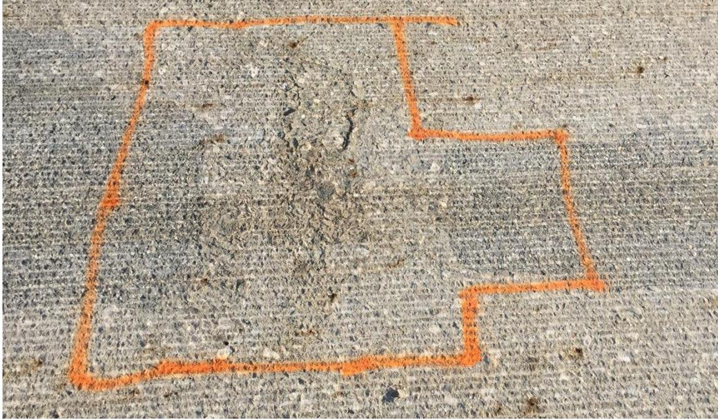
**Figure 3. Area marked for more in-depth removal**
