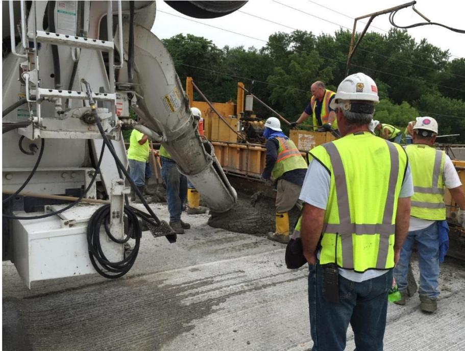
**Figure 6. Ready-mixed concrete being placed on the deck**
