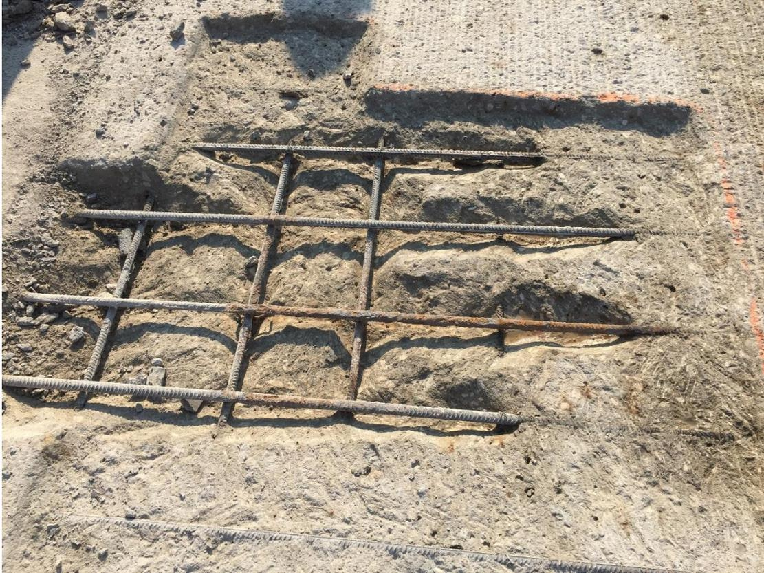
**Figure 5. Deteriorated area of the deck after removal of the substrate concrete**
