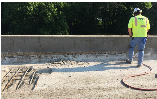
Concrete removed past the bottom of the embedded reinforcing steel (left side of image) and removal of concrete along barrier rail using jackhammer (right)
