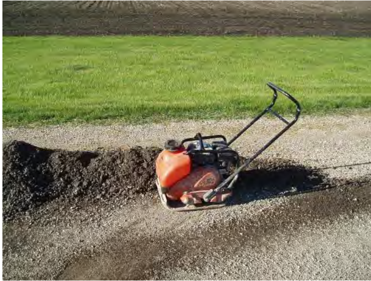
Figure 37. Longitudinal joint vibrating plate compactor
