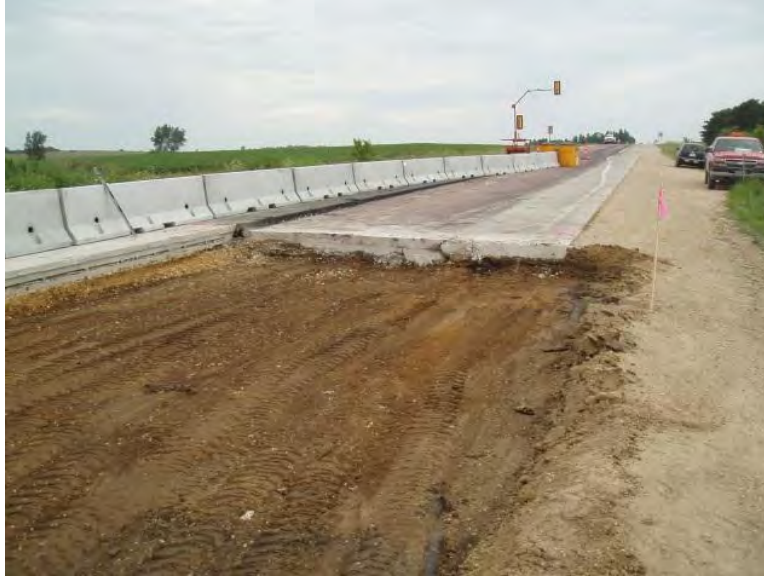
Figure 50. Pavement and shoulder strengthening removal
