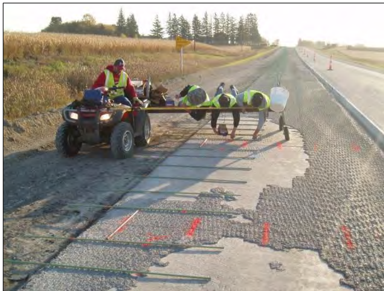
Figure 68. Tie bar clip automation
