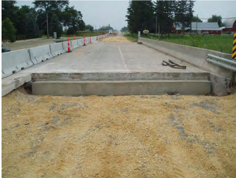
Figure 45. Paving notch replacement
