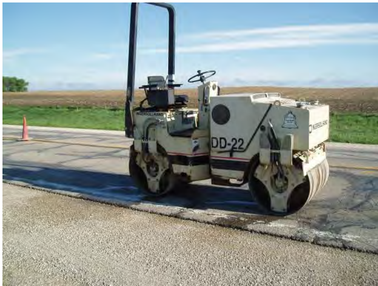
Figure 36. Longitudinal joint vibrating roller
