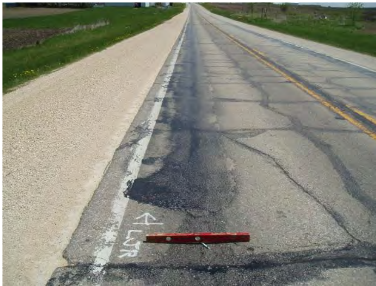
Figure 32. Longitudinal patch area
