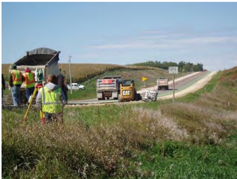
Figure 81. Dual total station control
