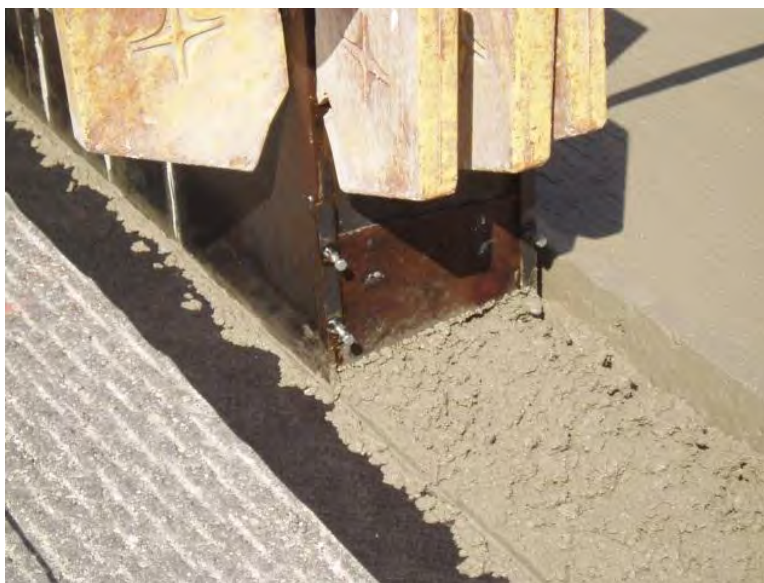
Figure 90. Centerline safety wedge extrusion gate
