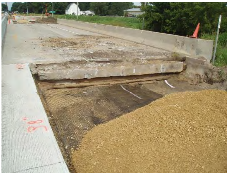
Figure 46. Bridge approach base preparation
