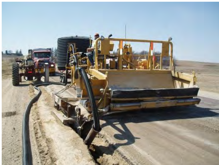
Figure 11. Subdrain installation
