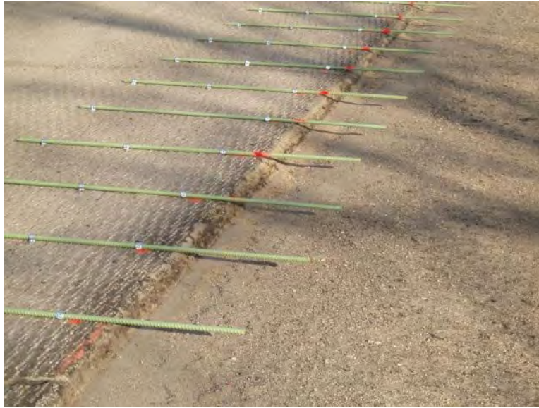
Figure 63. Widening final joint
