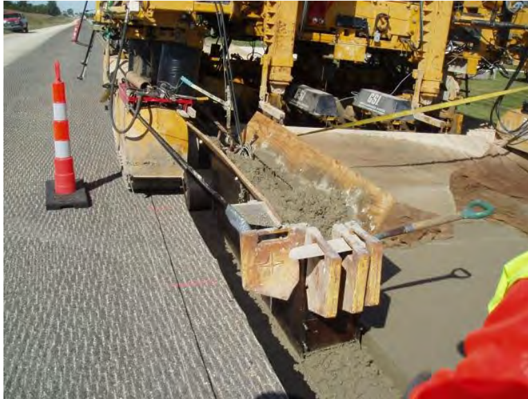
Figure 89. Centerline safety wedge slipform
