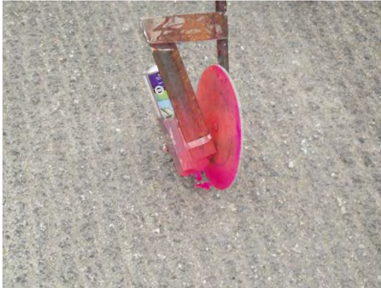
Figure 65. Tie bar location device
