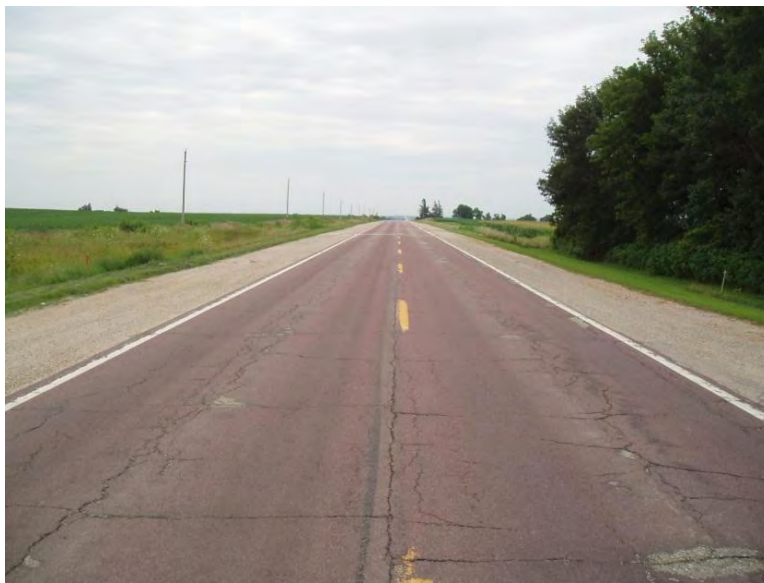
Figure 4. Existing pavement west end
