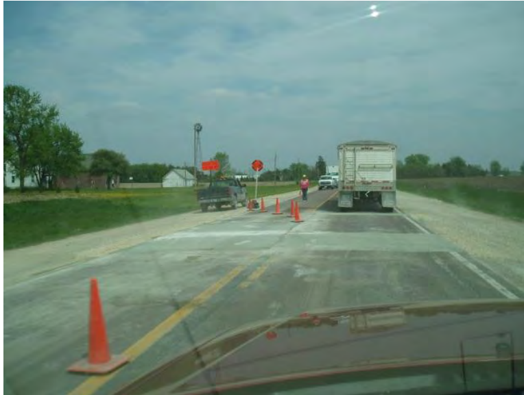
Figure 31. Patching lane delineation
