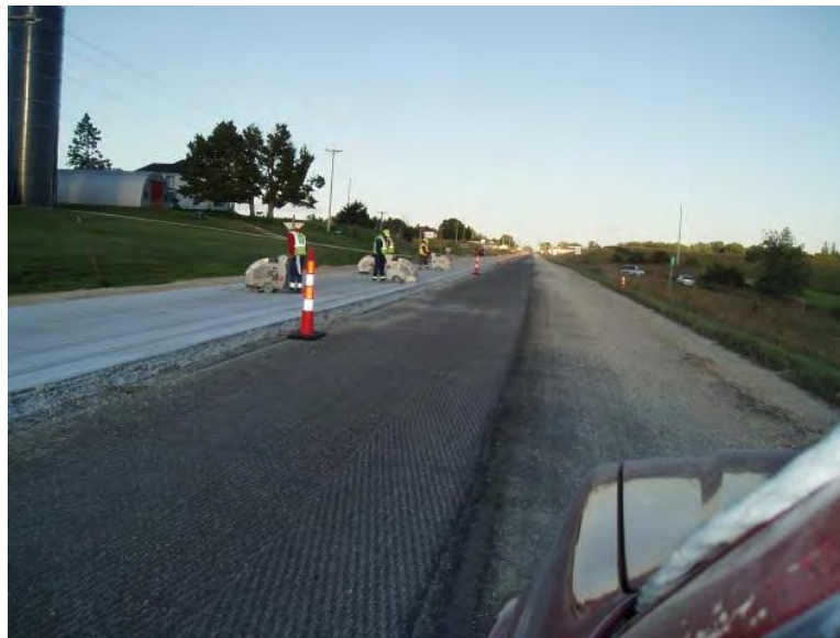
Figure 86. Transverse joint saws
