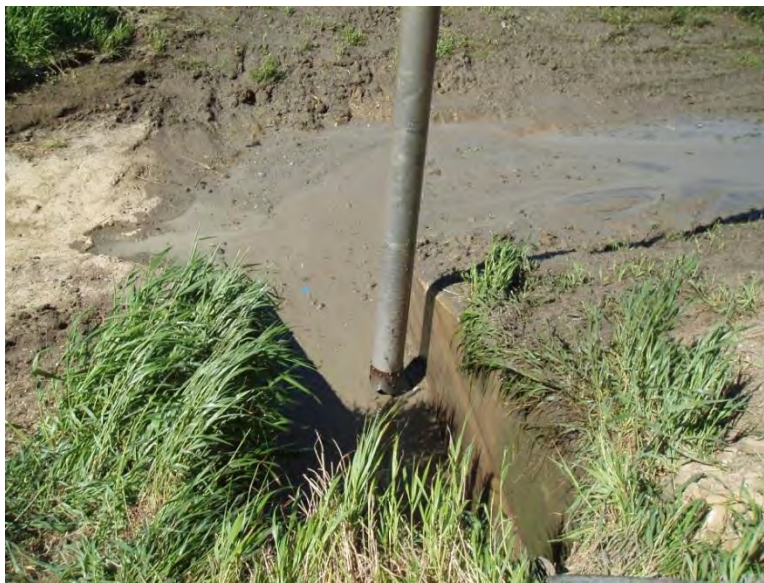
Figure 38b. RCB cleaning
