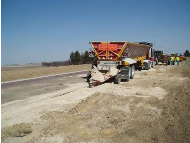
Figure 12. Granular backfill operation
