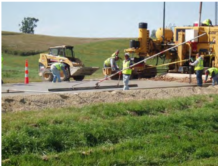
Figure 92. Centerline wedge concrete deposit
