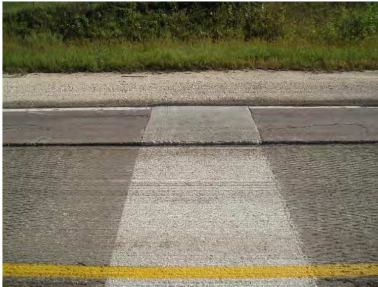
Figure 57. Milled PCC full-depth patch
