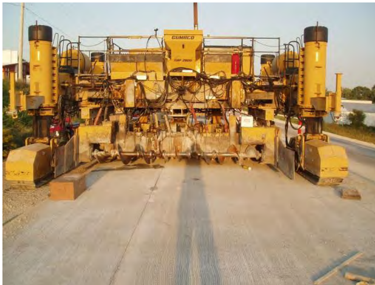
Figure 70a. Slipform paver
