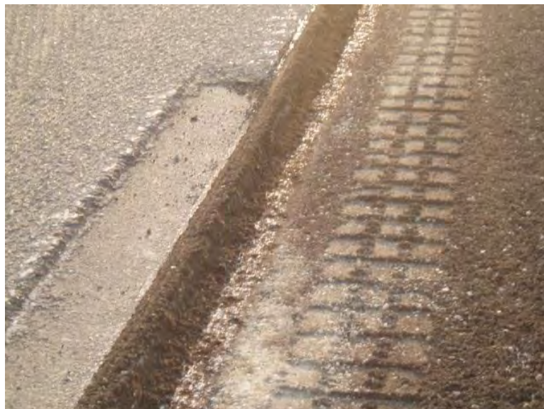
Figure 60. Milled widening unit area
