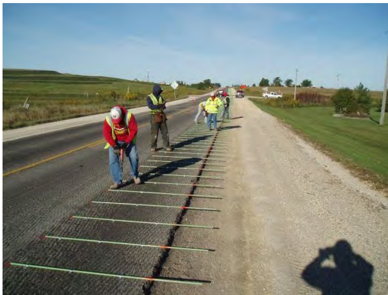
Figure 66. Tie bar installation
