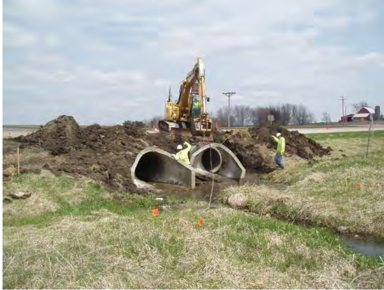
Figure 39a. Culvert extension/relay
