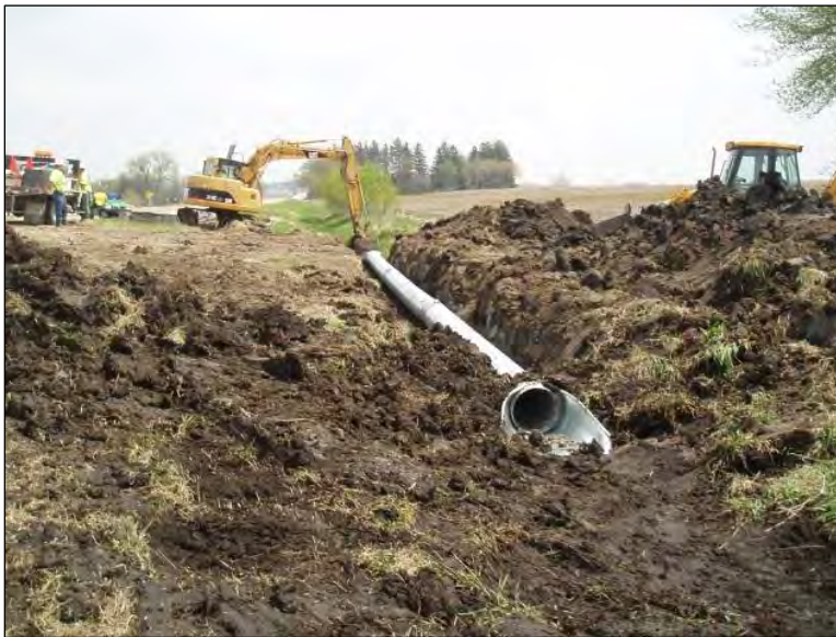
Figure 39b. Entrance pipe placement
