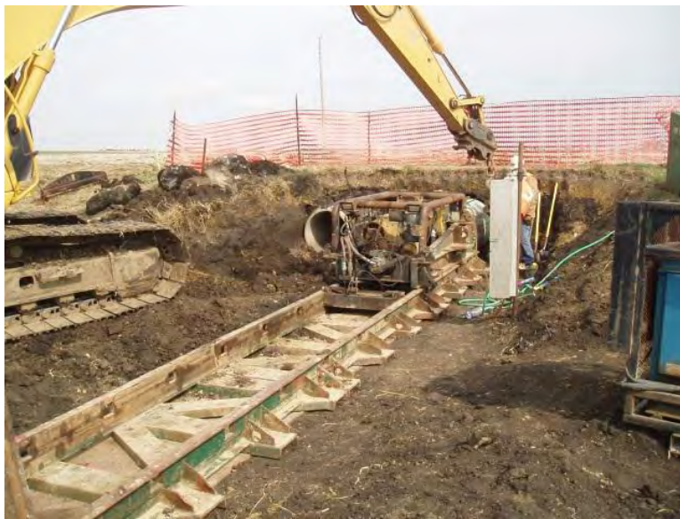
Figure 42. Culvert pushing pit
