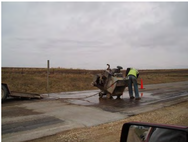
Figure 21. Sawing around patch area
