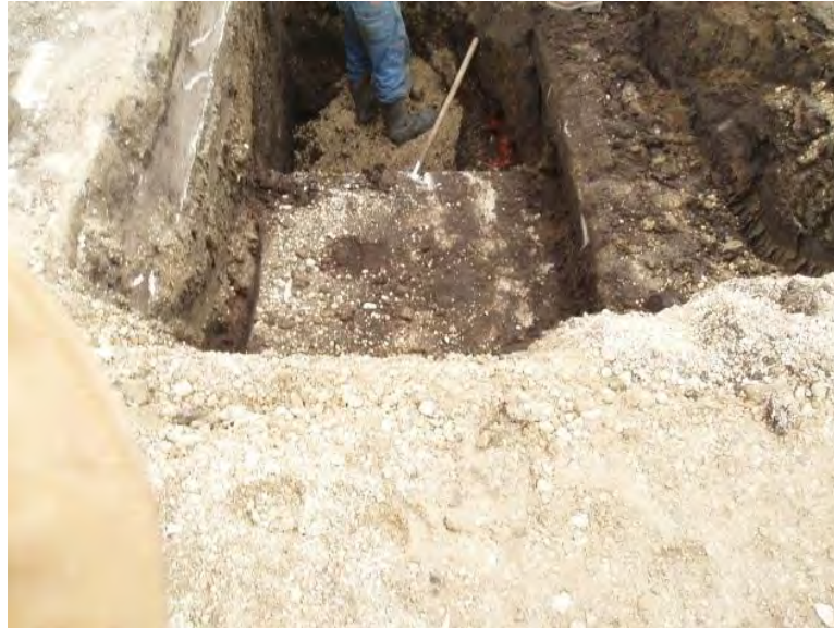
Figure 18. Existing subdrain repair
