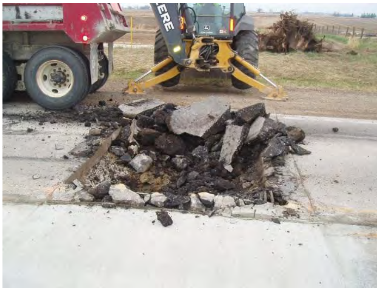
Figure 23. Patch area excavation
