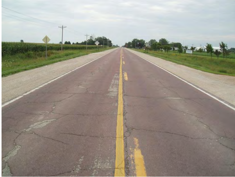
Figure 3. Existing pavement west end
