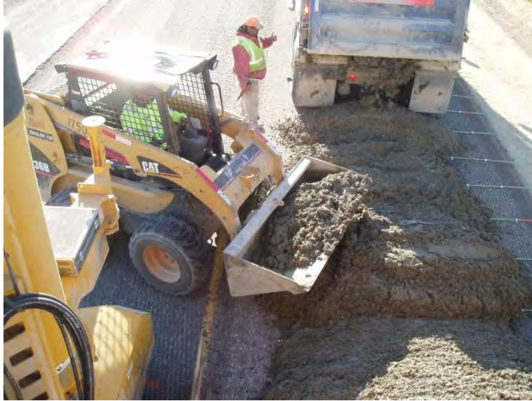
Figure 91. Centerline wedge concrete access
