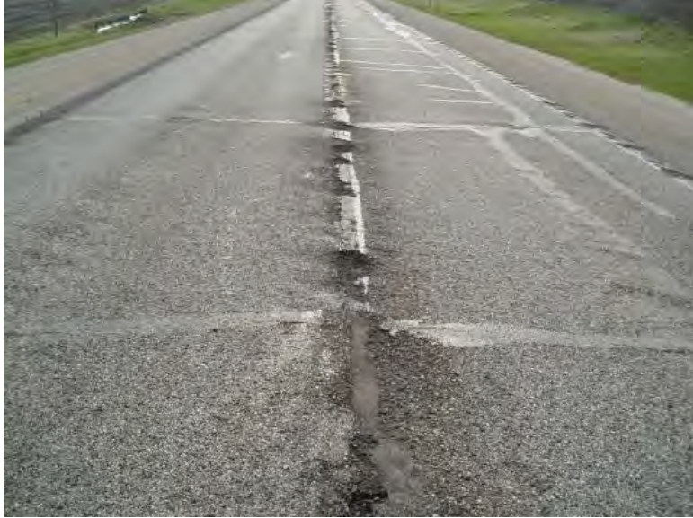
Figure 1. Existing pavement east end
