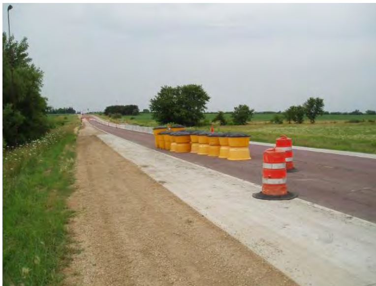
Figure 48. Temporary barrier traffic control
