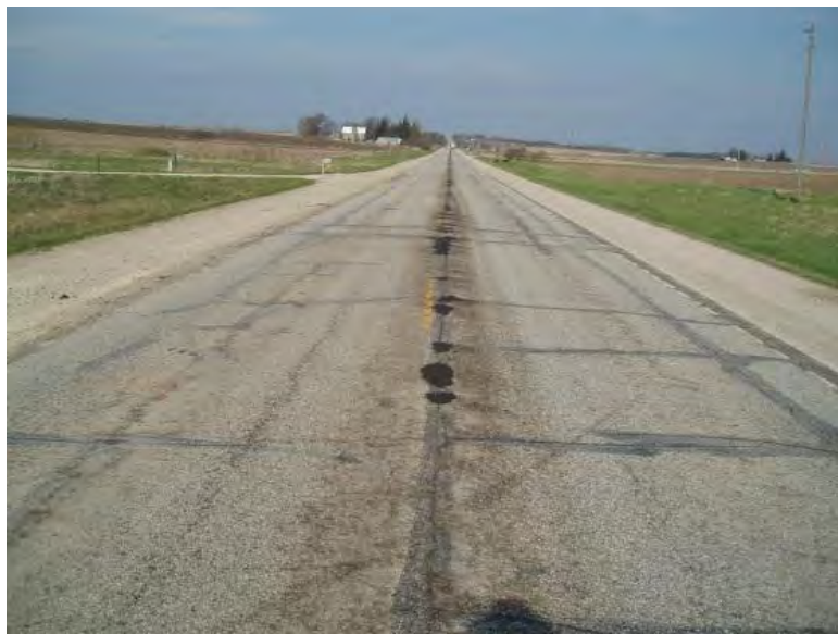
Figure 2. Existing pavement east end
