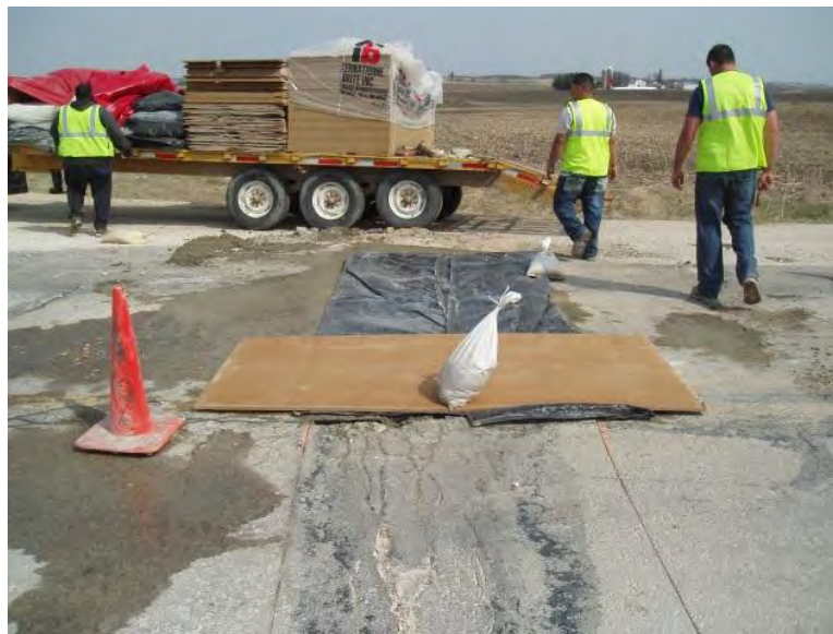
Figure 28. Patch curing
