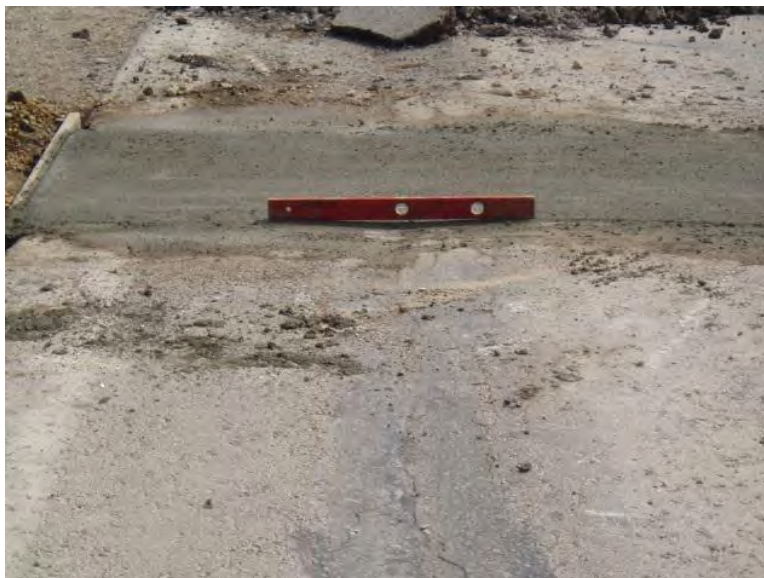
Figure 27. Full-depth patch surface finish
