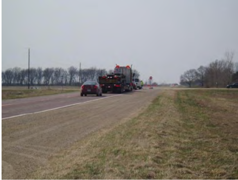
Figure 29. Patching traffic control
