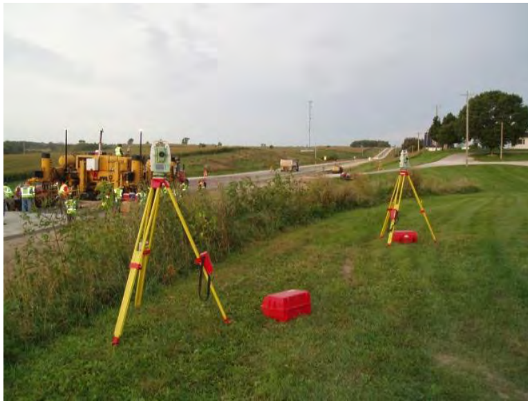
Figure 74. Robotic total station
