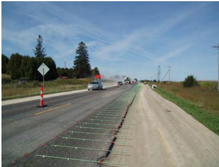
Figure 69. Pilot car operation
