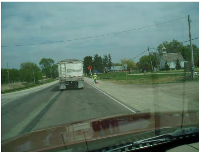
Figure 30. Patching flagger station
