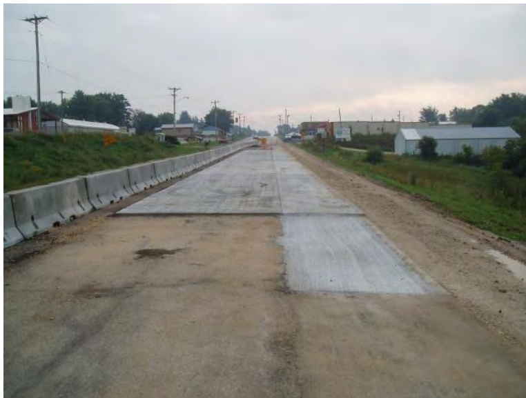
Figure 43. EOP transition section
