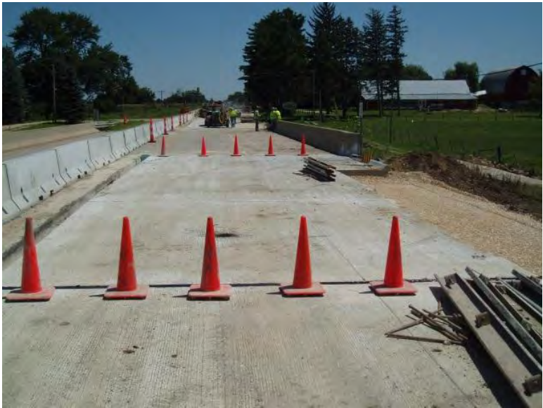
Figure 97. Bridge #1 EBL transition
