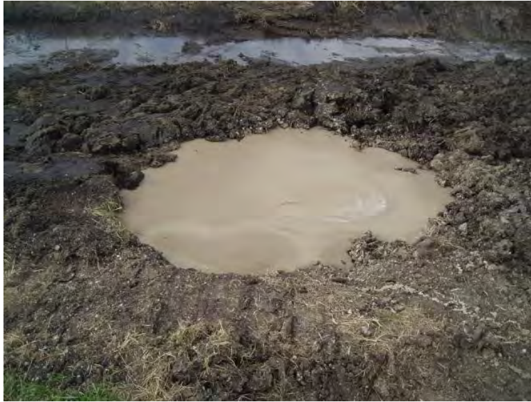
Figure 40. Culvert plugging
