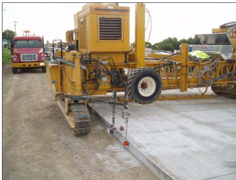
Figure 73. Cure/texture machine guidance control
