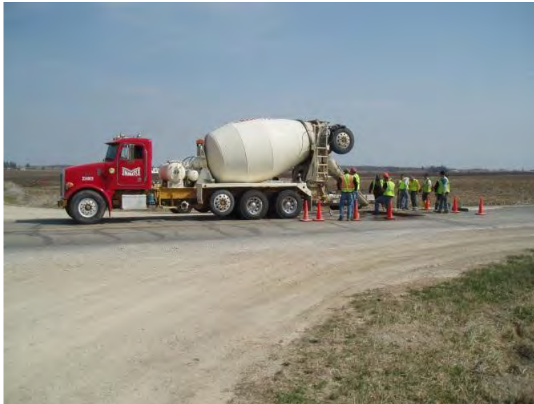
Figure 26. Concrete delivery for patches
