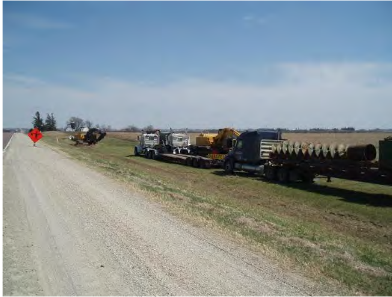
Figure 41. Culvert pushing equipment
