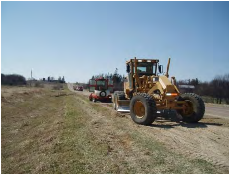
Figure 13. Subdrain trench finishing
