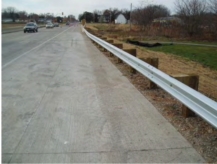
Figure 47. Paved bridge shoulder
