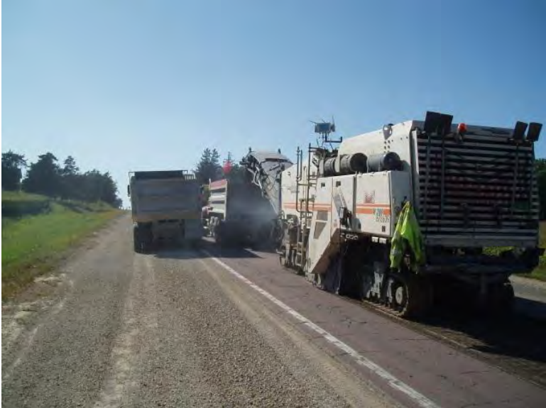
Figure 54. Milling to grade, pass #1
