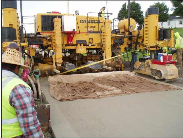
Figure 70b. Slipform paver burlap drag
