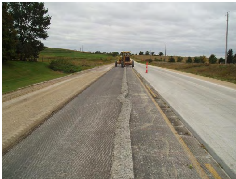
Figure 94. Centerline wedge removal
