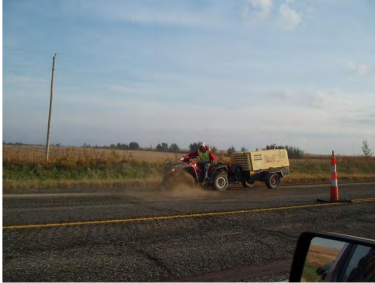
Figure 61. Widening edge cleaning
