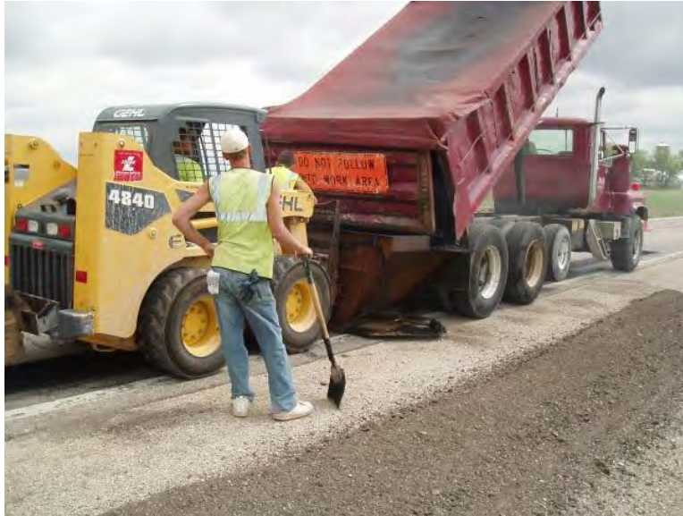
Figure 35. Longitudinal patch filling
