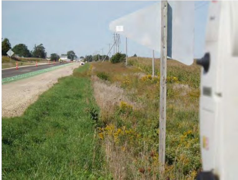
Figure 79. Prism 3 Site (near second power pole)
