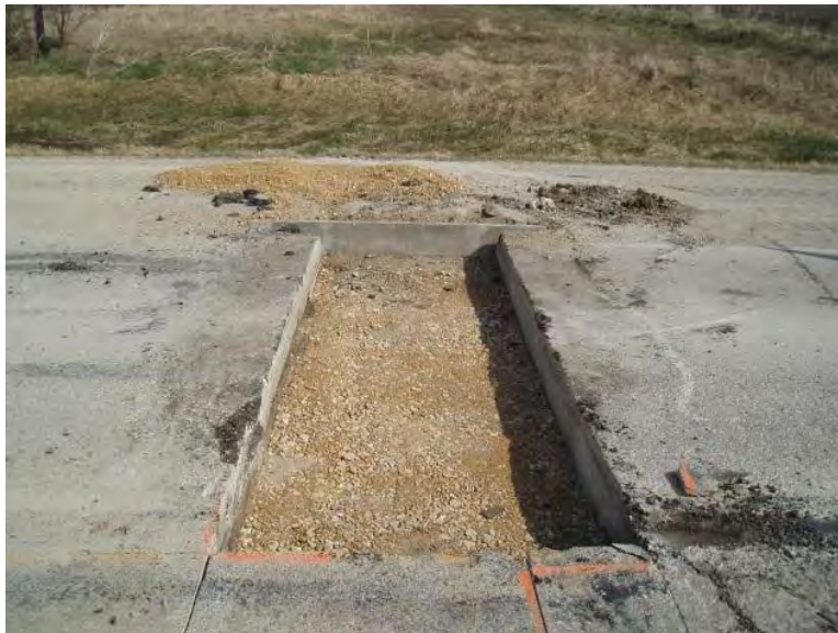
Figure 25. Compacted patch area subgrade
