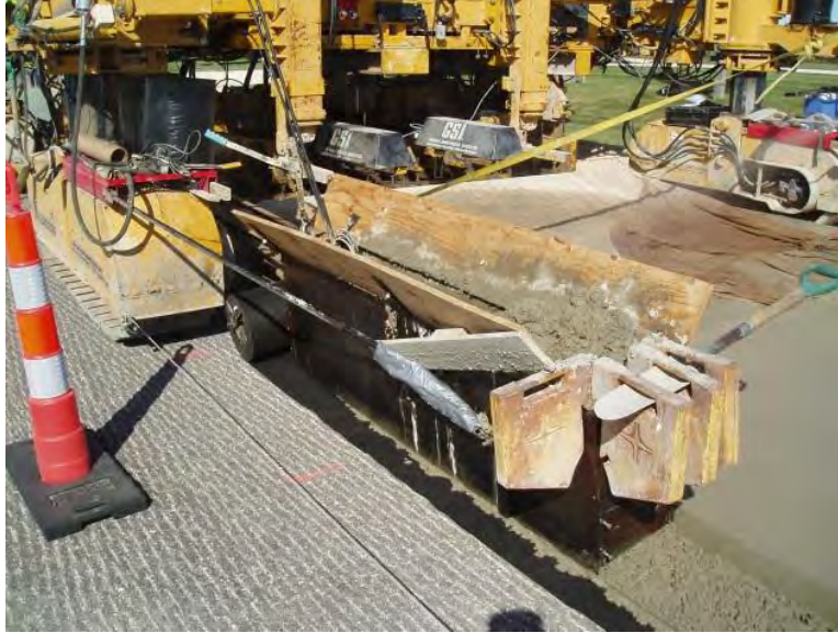
Figure 93. Centerline wedge bond breaker applicator
