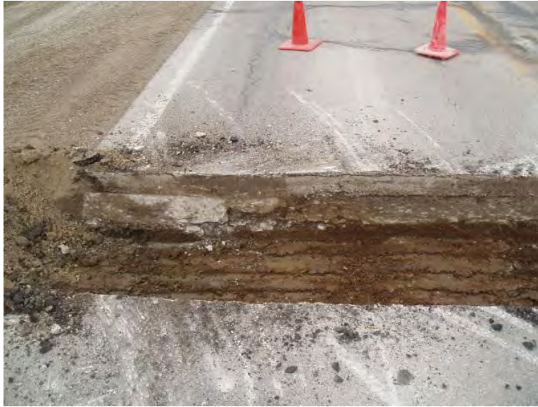
Figure 24. Completed patch excavation
