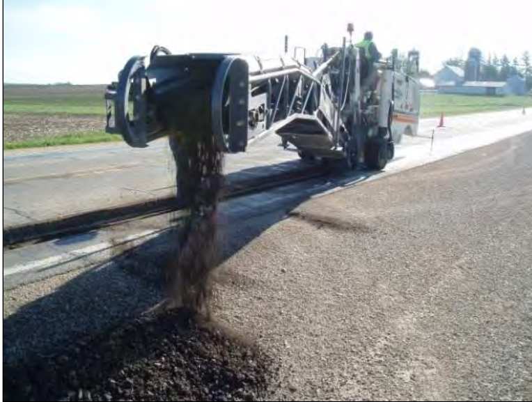
Figure 33. Longitudinal patch removal milling
