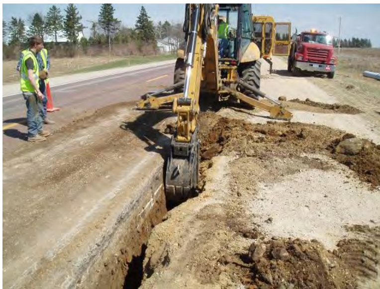
Figure 17. Subdrain boulder removal
