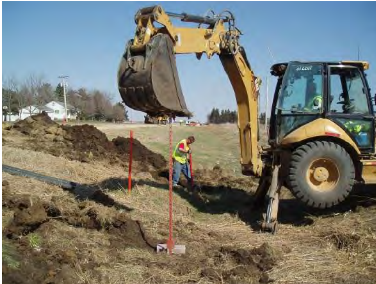
Figure 15. Subdrain outlet excavation
