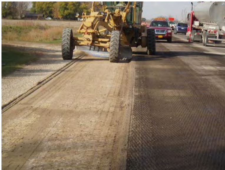
Figure 62. Slipform padline preparation
