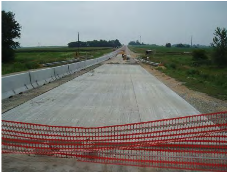
Figure 44. Bridge transition section
