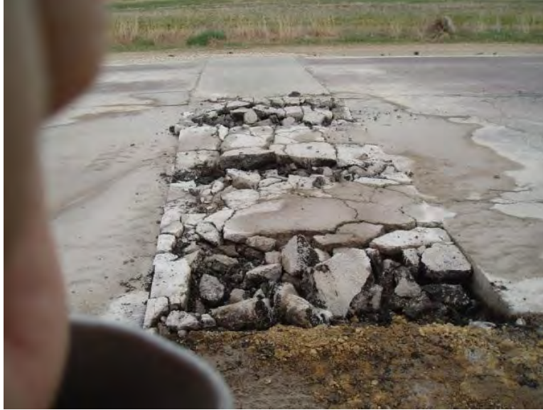
Figure 22. Patch area demolition
