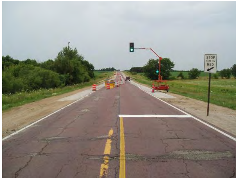
Figure 49. Shoulder strengthening in place
