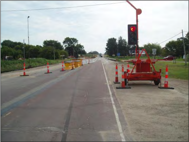
Figure 96. BOP Bridge #1 traffic control
