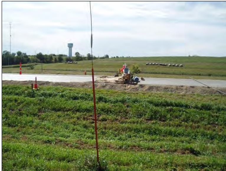
Figure 71. Workbridge and burlap drag
