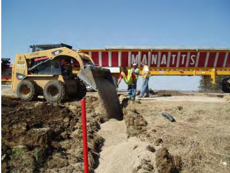
Figure 16. Subdrain outlet backfilling
