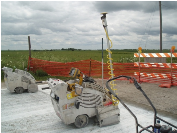
Figures 4 & 5. Standard Concrete Saw Outfitted with GPS Unit
