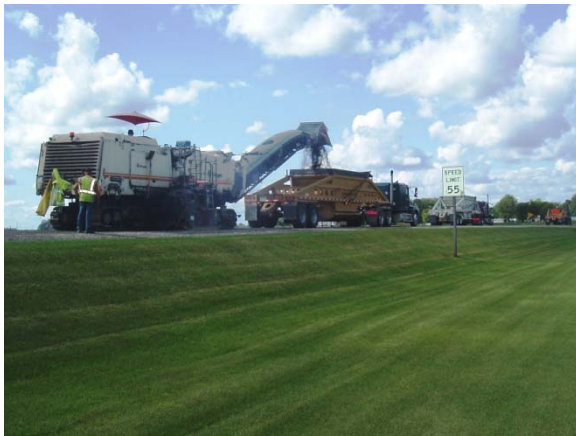
Figure 6. Mainline Pavement Milling
