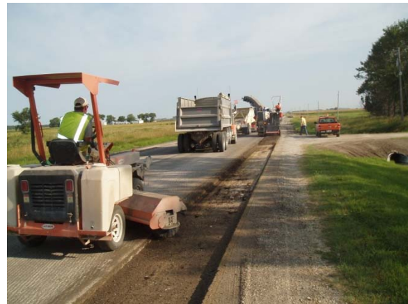
Figure 7. Shoulder Milling for Pavement Widening
