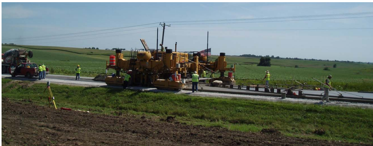
Figure 3. Dual Lane Stringless Paving Operation
