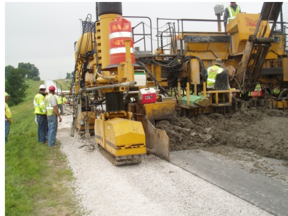
Figure 2. Slipform Paver Utilizing Stringless Paving
