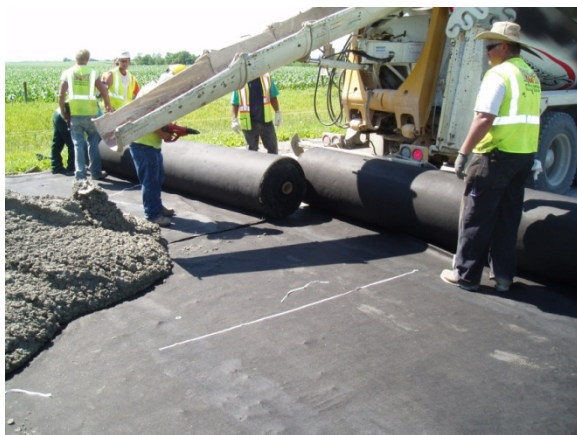
Figure 8. Geotextile Bond Breaker between Paver and Ready Mix Trucks
