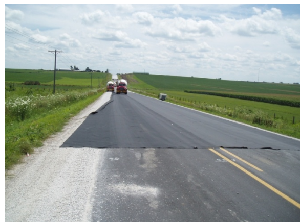
Figure 9. Equipment Operating over Geotextile Bond Breaker
