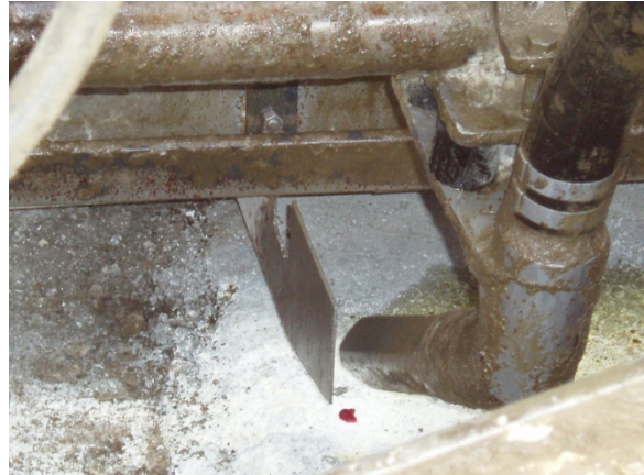
Figure 14. Longitudinal Joint “Knife” Installed on Slipform Paver
