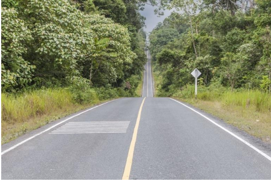
Figure 2. Example of transverse rumble strips
