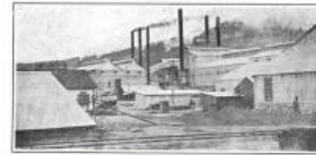
CEMENT PLANT AT MONOLITH.
