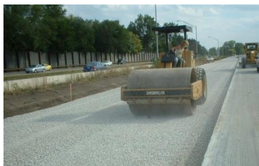
Figure 5. Unstabilized aggregate subbase
