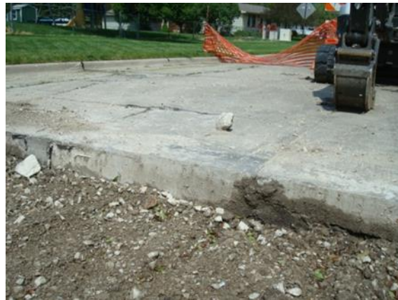
Figure 24. Moist subgrade conditions
