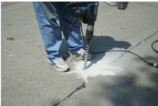
Figure 20. Drilling prior to DCP test
