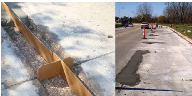
Figure 5-2. Milled joint for removal of spalling (left photo) and finished PDR (right photo, courtesy of City of West Des Moines, Iowa)
