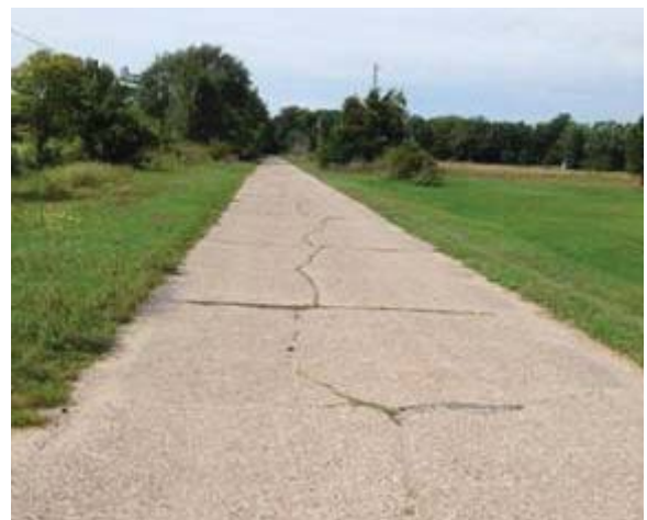
Figure 1-2. Moscow street in 2014 (photo courtesy of Kurt Smith, Applied Pavement Technology, Inc.)
