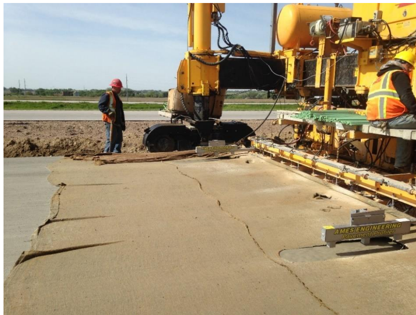
Figure 9. Paving on I-80 in Lincoln, NE
