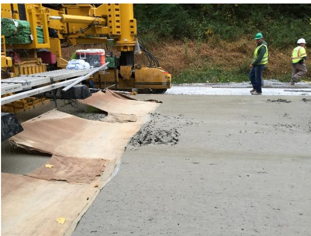
Figure 5. Isolated Areas of Mixture Exhibited Poor Finishing Characteristics
