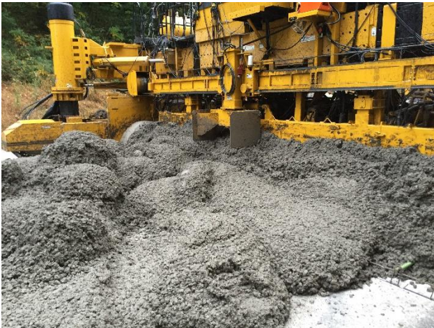
Figure 3. Concrete Placement at the Front of the Paver
