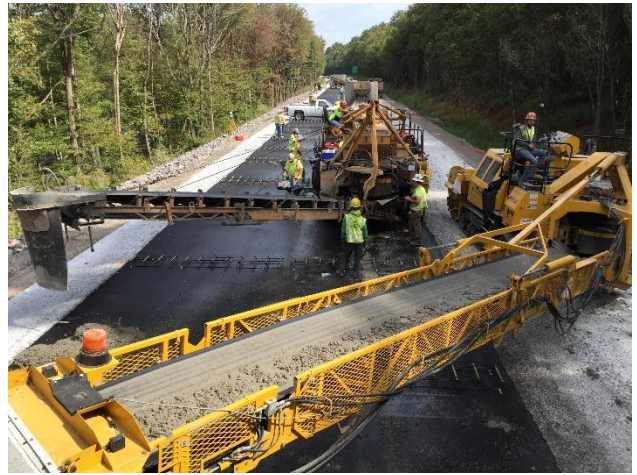
Figure 2. Concrete Spreading by Placers Ahead of the Slipform Paver
