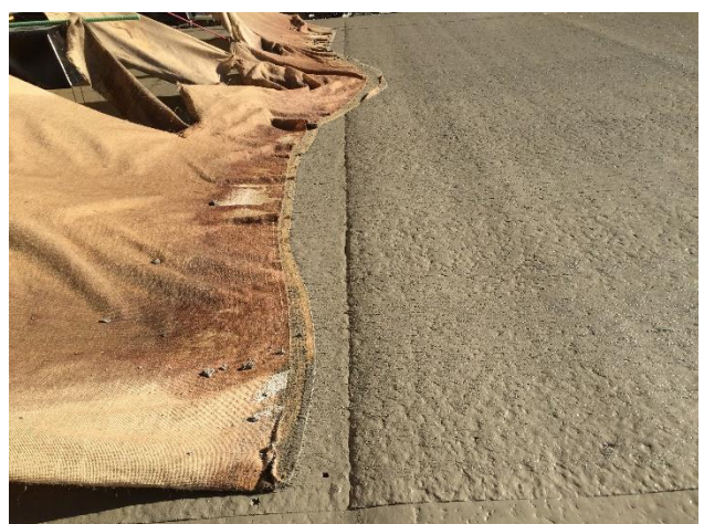
Figure 6. Close-up of Profile Feature Created by a Paver Stop (mitigated by hand finishing)
