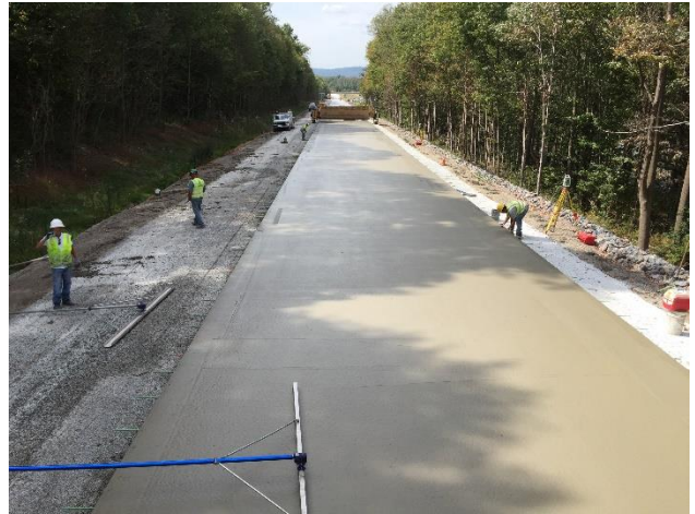
Figure 4. Typical Hand Finishing Behind the Paver
