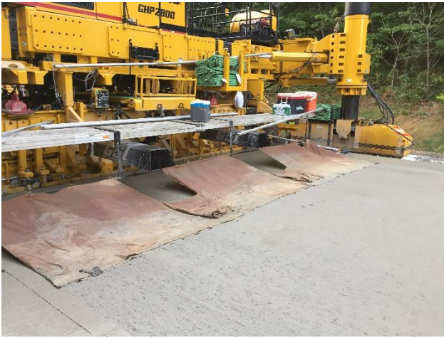
Figure 1. Gomaco GSI Mounted to 2800 Paver
