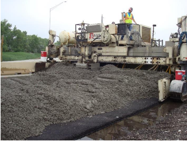
Figure 3. Concrete distribution in front of the paver.
