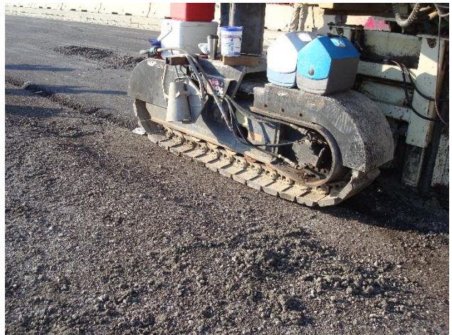
Figure 6. Stable padline on the non-companion paving side.
