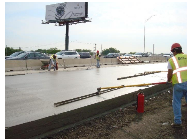
Figure 8. Typical Hand Finishing Behind the Paver
