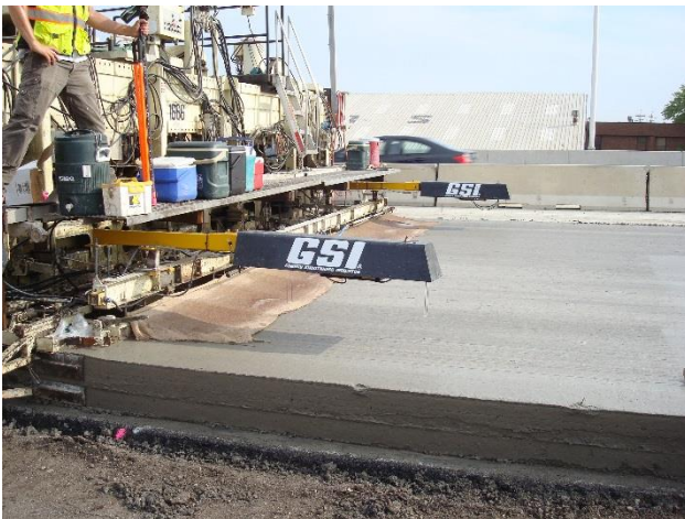
Figure 1. Gomaco GSI behind finish pan and burlap.
