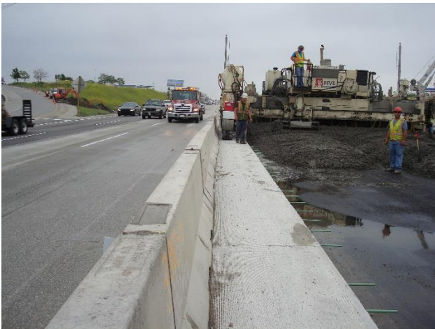
Figure 5. Constrained paving conditions on the companion paving side.
