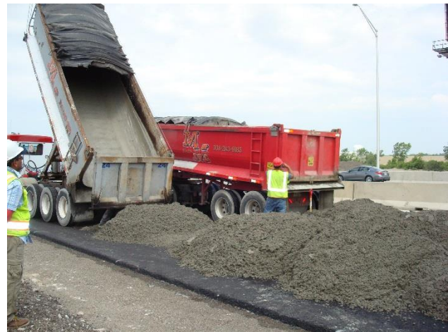
Figure 2. Concrete delivery to the paver.
