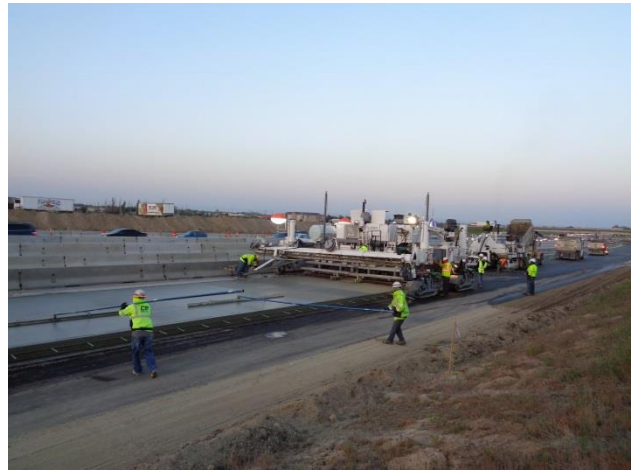
Figure 4. Use of a Final Finisher (auto-float) and Hand Finishing Behind the Paver
