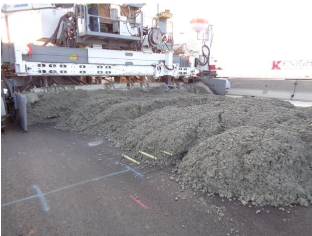
Figure 3. Concrete Deposited on Dowel Baskets Ahead of the Paver
