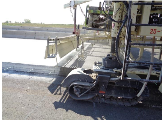
Figure 6. Application of Curing Compound
