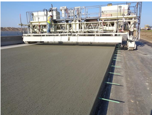
Figure 5. Artificial Turf Drag and Longitudinal Tining
