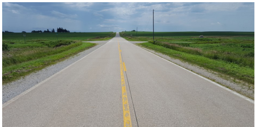
Grundy County Highway T-55 with 6-inch overlay in 1978
