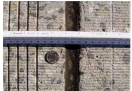
**Figure 5. CPSCP Section 209-D having large within-section variability with measured OBSI level versus distance using long and short averaging lengths (left) and photo of pavement joint corresponding to significant tire-pavement noise generation (right)**
