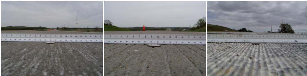
Figure A-1. Photographs of typical drag, timing, and diamond grinding textures.
