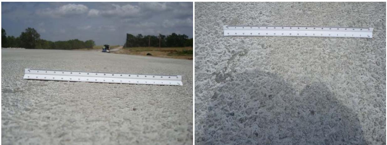
Figure 3: Surface B – Exposed Aggregate.
