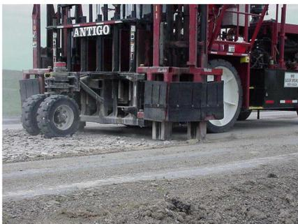
Figure 1. Rubblization of Concrete Surface
